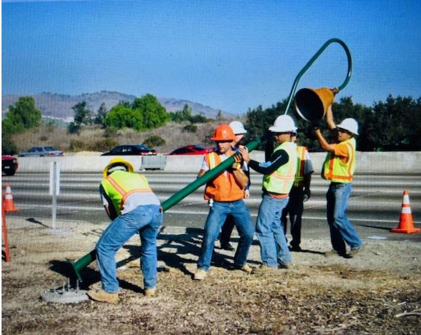
Figure 6: Caltrans workers installing an El Camino Road Marker in 2004. (Photo courtesy of SCMSHP).
