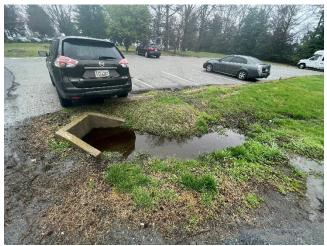
Figure 19: Ponding area at the end of the swale after a rain event (Ren)
