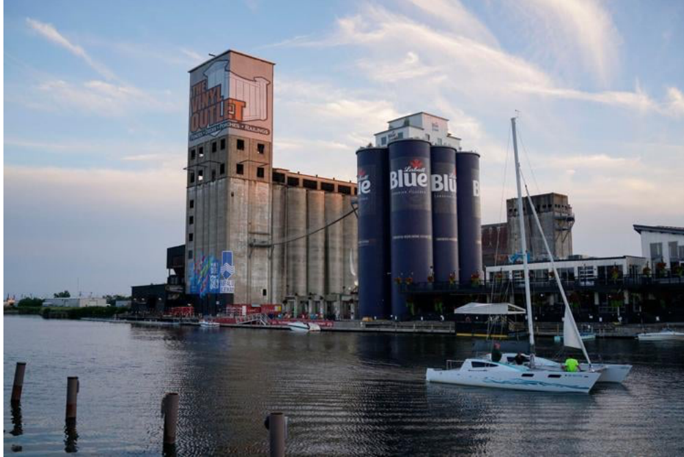
Figure 4.1. The “6 Pack” Silo’s at Buffalo River Works Campus. July 30, 2020. The Buffalo News https://buffalonews.com/news/local/article_fdf5fb38-d101-11ea-a556-1b7fbdc083a.html .
