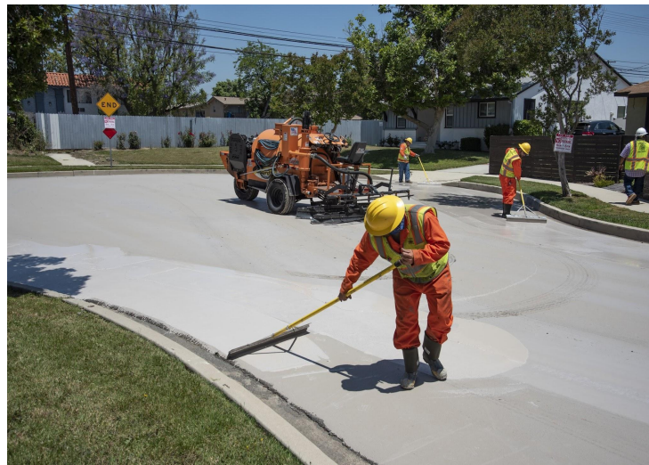
Figure 65: A construction worker in Los Angeles applying cooling paint to a residential road.
