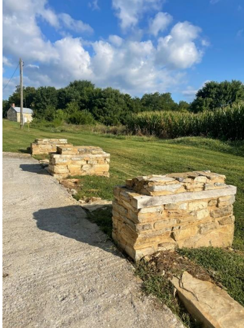
Figure 27. Roulette Barn, corn crib/wagon shed piers. (Tabitha Gold, 2022).
