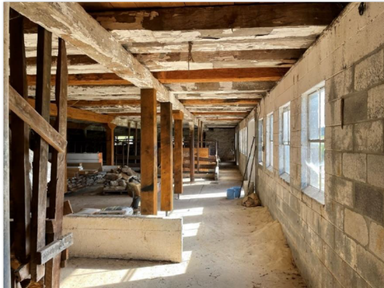
Figure 50. Post and Beam replacements near CMU wall (Tabitha Gold, 2022).
