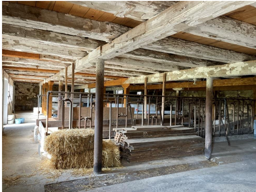
Figure 41. Hollow metal poles added ca 1950's by the Roulette Family. (Tabitha Gold, 2022).
