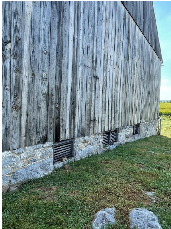
Figure 36. Roulette Barn, Foundation Walls With Vents. (Tabitha Gold. 2022).
