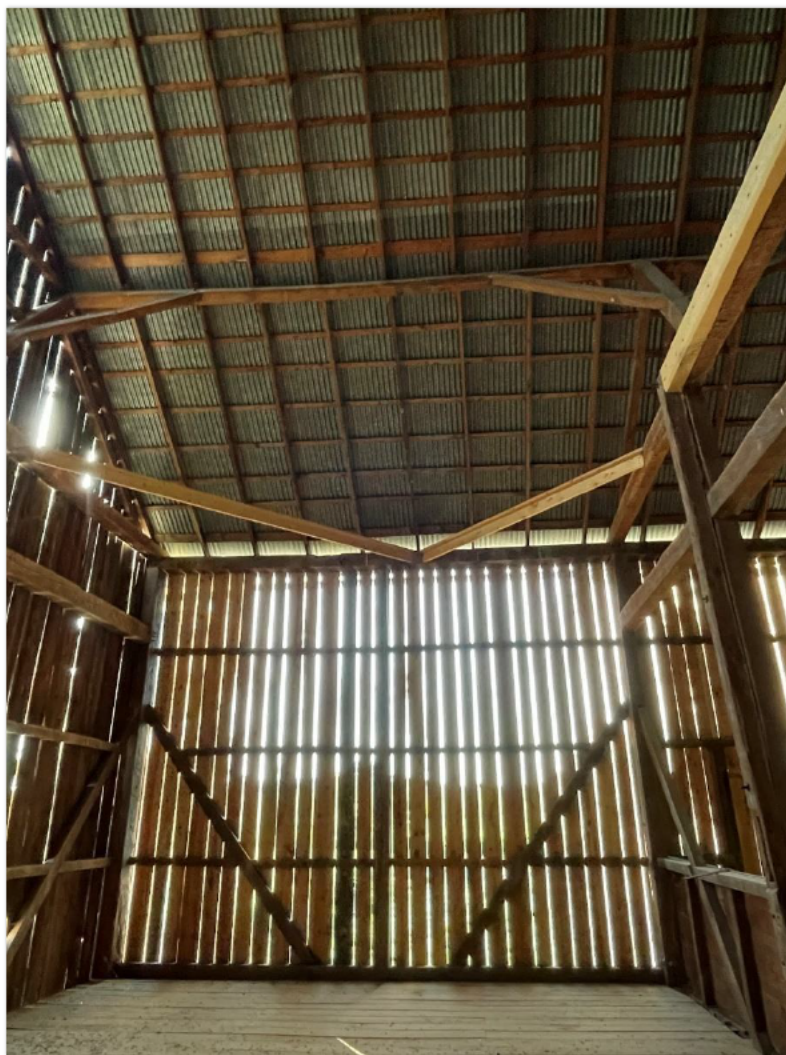
Figure 18. Roulette Barn down braces connecting from corner post to sill. (Tabitha Gold 2022).
