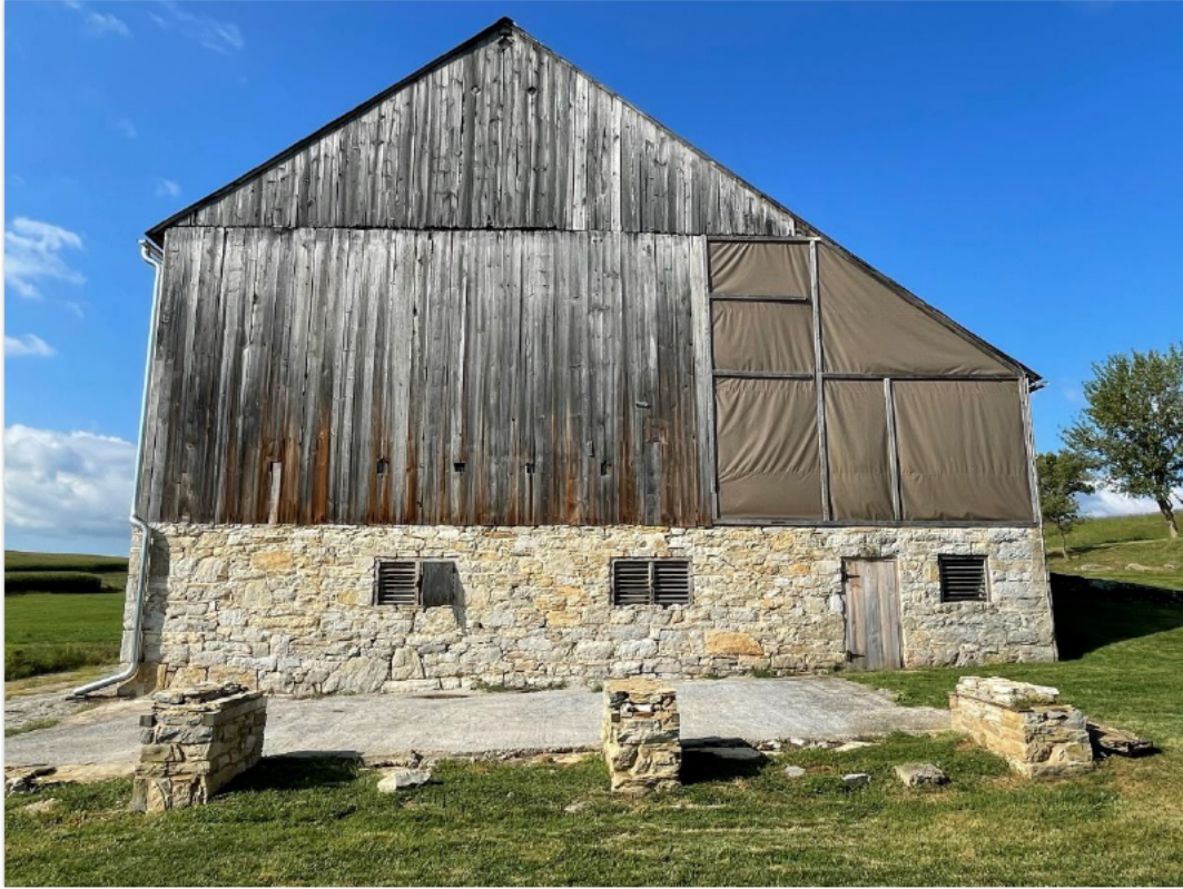
Figure 38. Corn crib/wagon shed stone piers. (Tabitha Gold, 2022).
