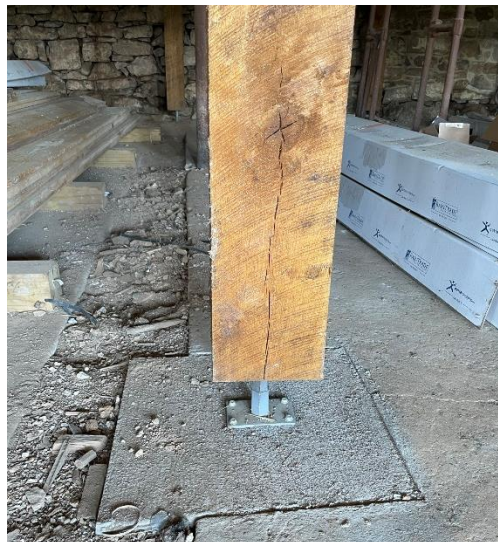
Figure 44. Post replacement under the summer beam on the lower lever (Tabitha Gold, 2022).
