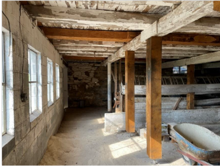
Figure 49. Post and beam replacements previously performed by NPS in the 2018 repair project (Tabitha Gold, 2022).
