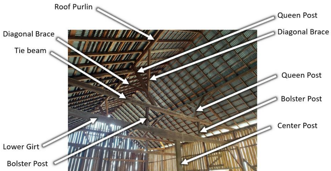
Figure 10. Bolster Posts Connecting Tie Beam (Tabitha Gold, 2022).
