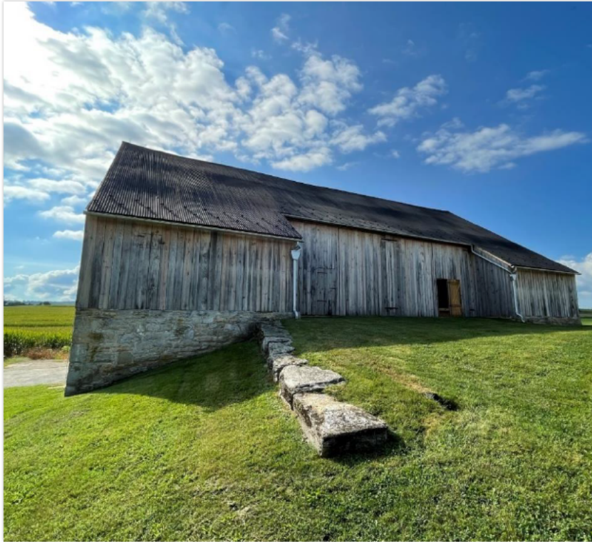
Figure 16. Roulette Barn, bank side showing earthen ramp and outsheds. (Tabitha Gold 2022).
