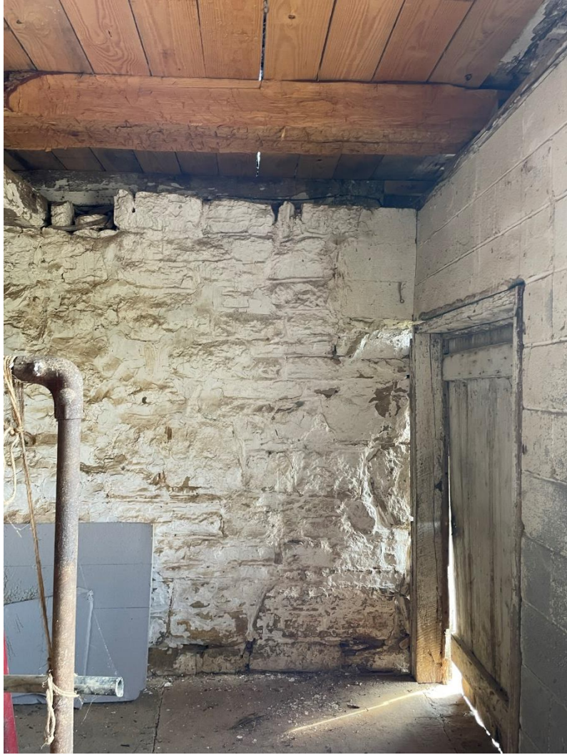
Figure 42. Viewpoint of CMU wall intersecting with limestone foundation wall (Tabitha Gold 2022).
