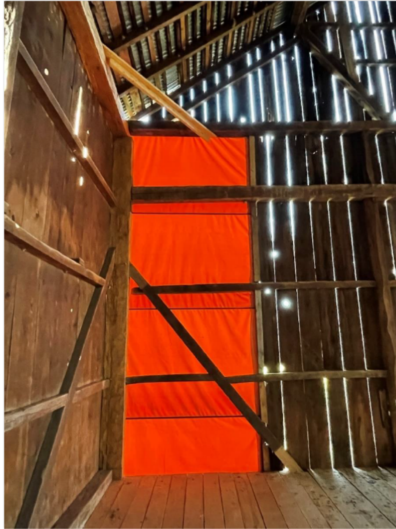
Figure 19. Roulette Barn, down braces on east gable wall. (Tabitha Gold, 2022).
