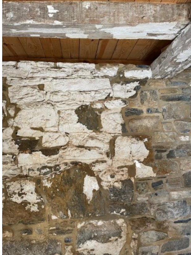
Figure 26. Roulette Barn, Whitewash remnants on stone foundation wall (Tabitha Gold, 2022).
