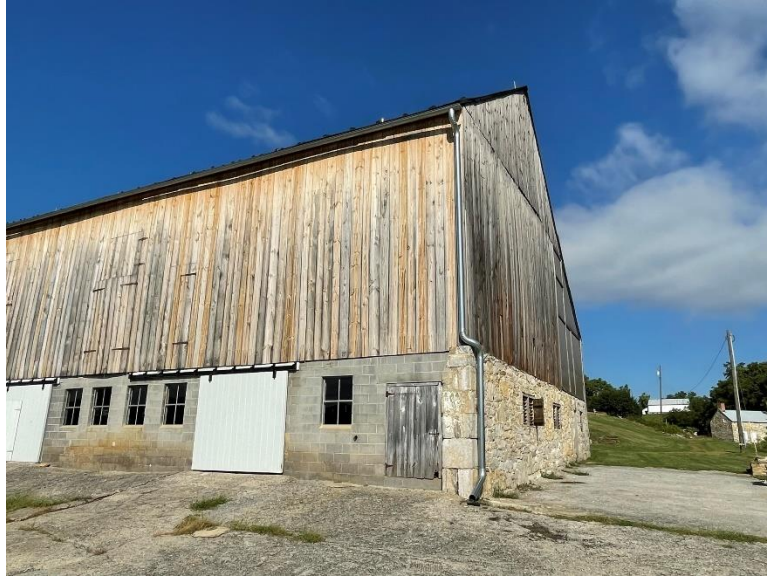
Figure 43. Exterior showing CMU wall intersecting with limestone foundation wall (Tabitha Gold, 2022).
