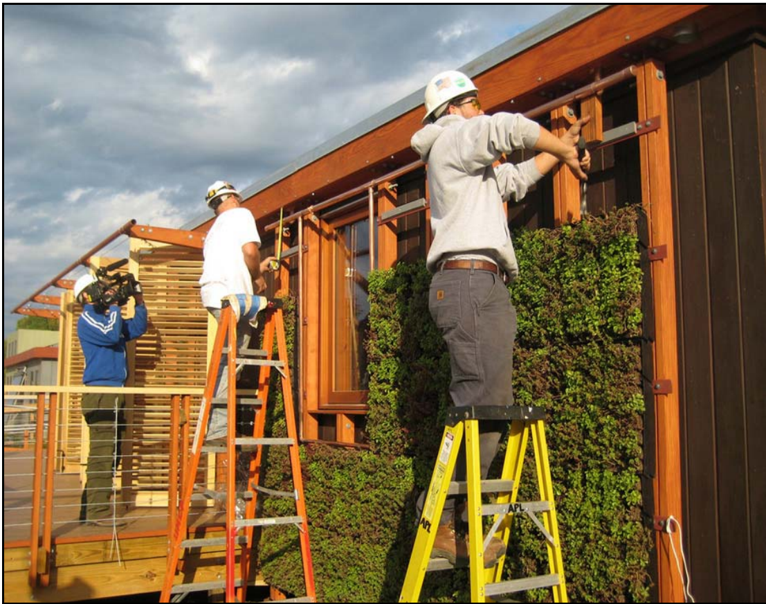
Figure 95. Installation of the Rainwater Filtration System
