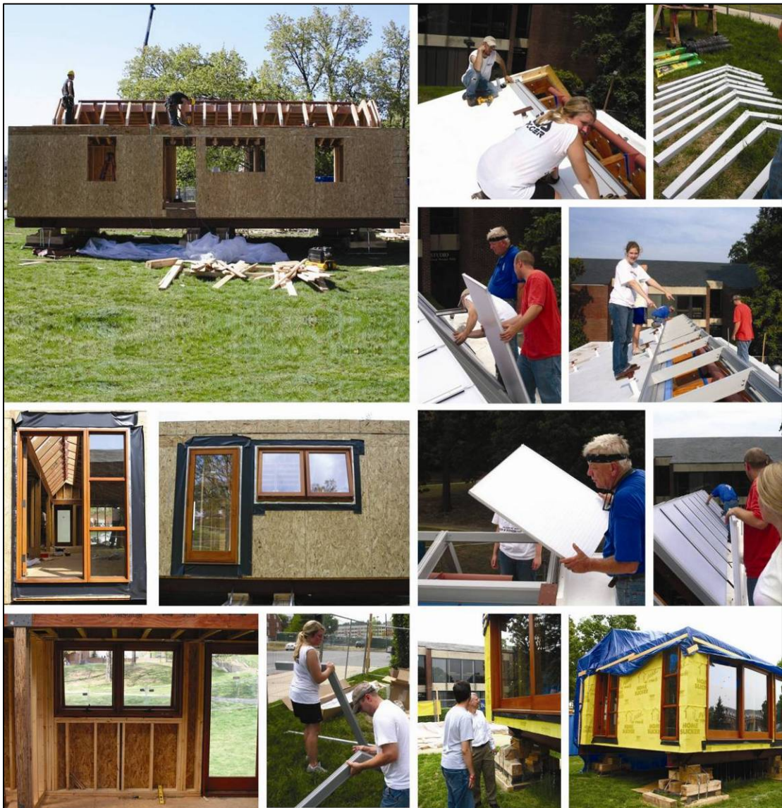
Figure 78. Door and Window Installation.
