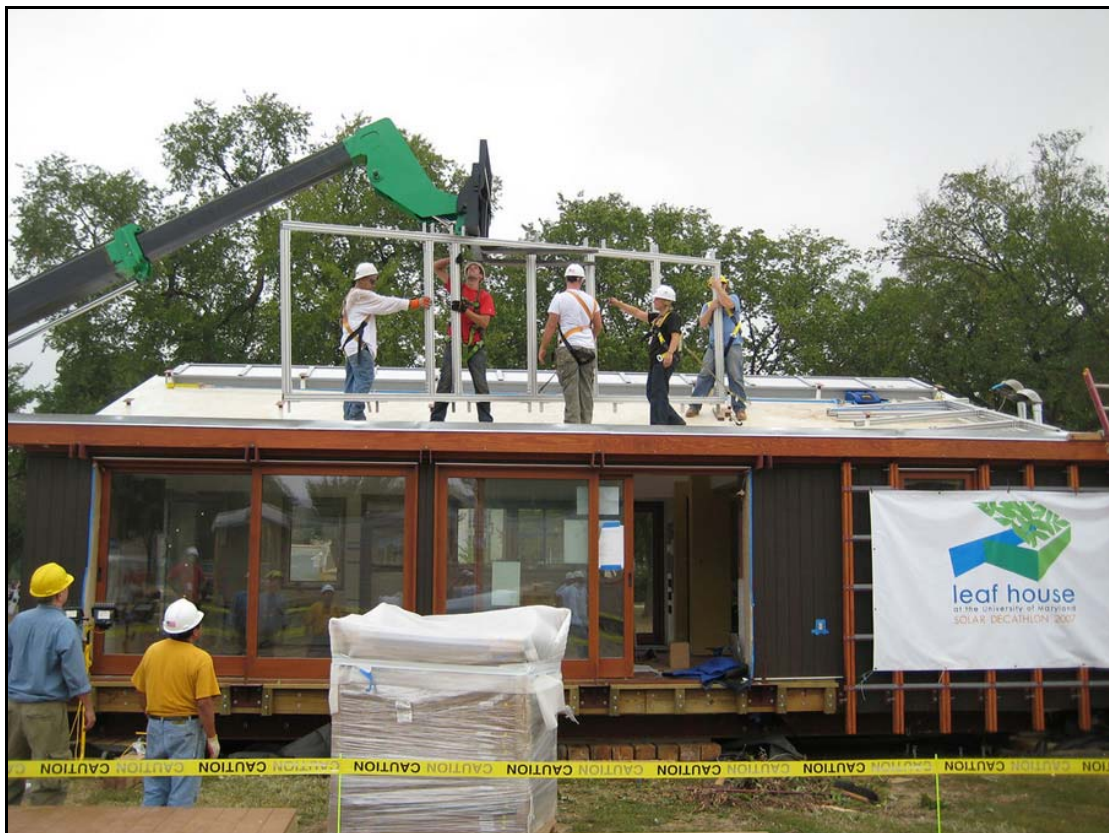
Figure 94. Reassembly of the PV Racking System
