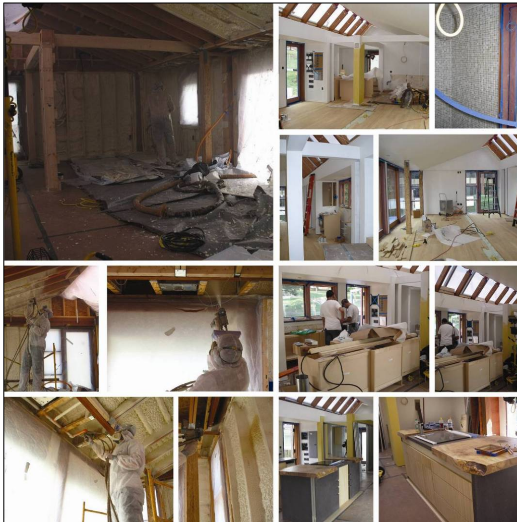
Figure 86. Insulation and Finishes Installation.
