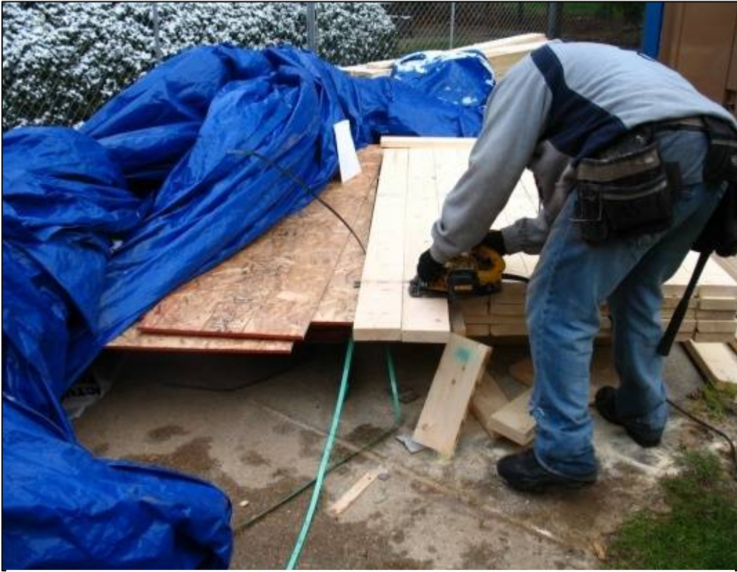
Figure 4. Cutting of FSC 2"x6" Studs for Wall Framing
