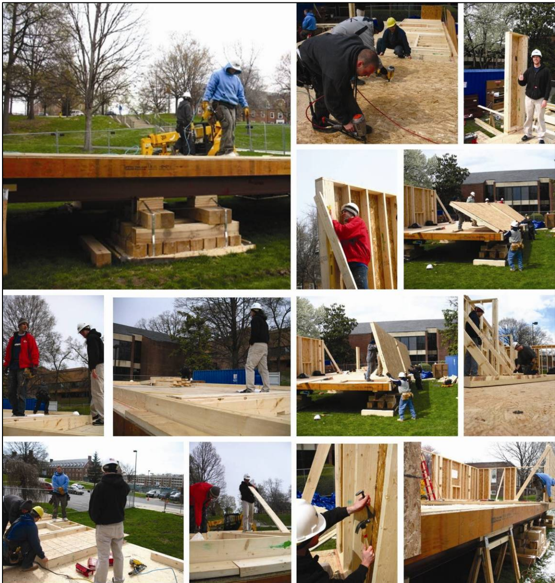
Figure 74. Wall Construction.
