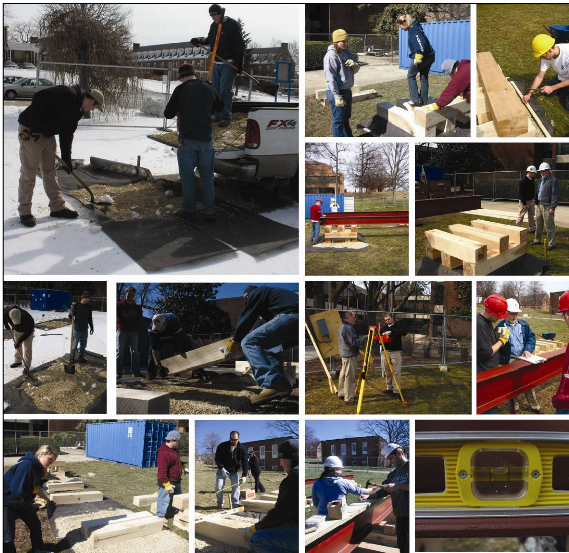
Figure 72. Foundation Sequence.
