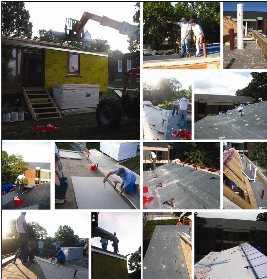
Figure 82. Finish Roof Installation.
