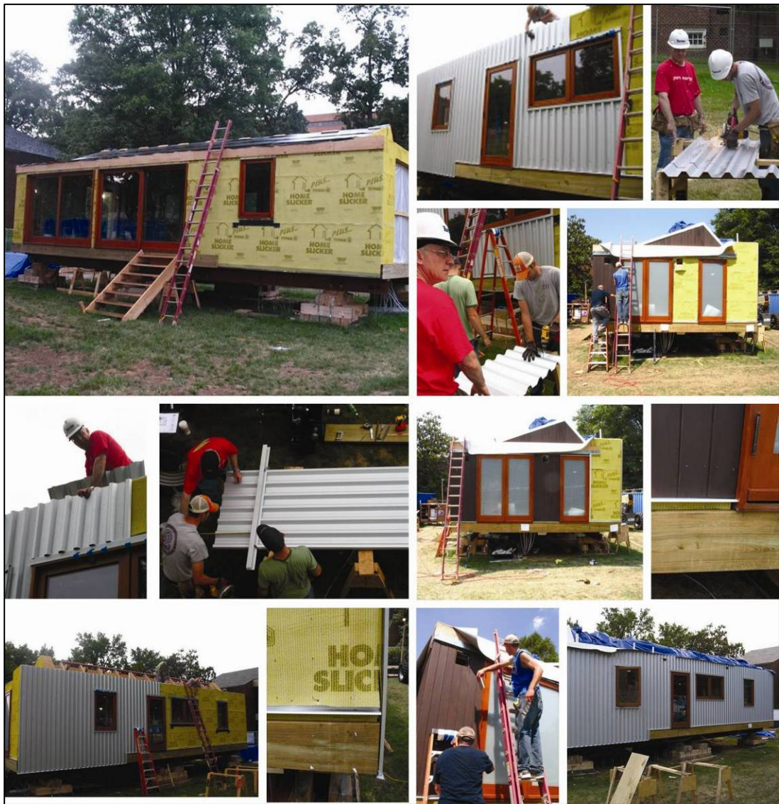
Figure 80. Siding Installation.
