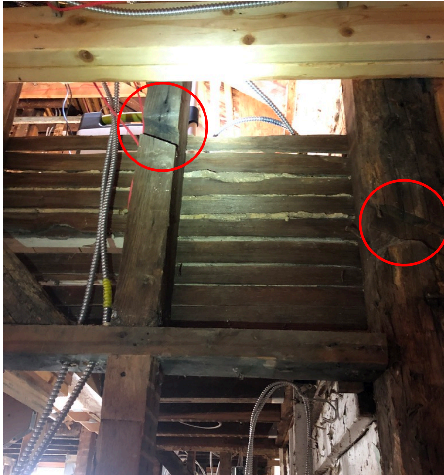
Figure 53. Evidence of a no longer extant “let-in” brace in the Phase Four addition appended to the original dwelling, which provides physical evidence that this section was constructed using balloon framing techniques. (Source: Francesca Evans, 2022)
