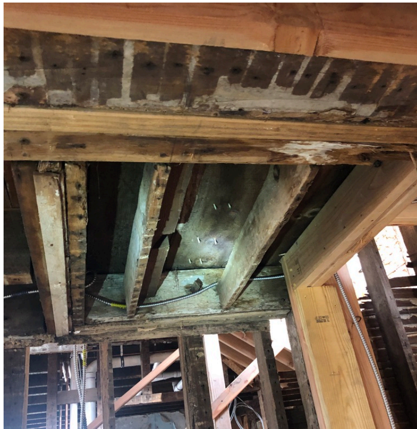
Figure 25. Framing evidence of a small opening providing access to the garret in the half-story. (Source: Francesca Evans, 2022)
