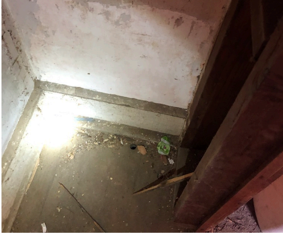
Figure 30. Tongue and groove floorboards and trim in the closet. These floorboards run east to west while the original flooring runs north to south. (Source: Francesca Evans, 2022)
