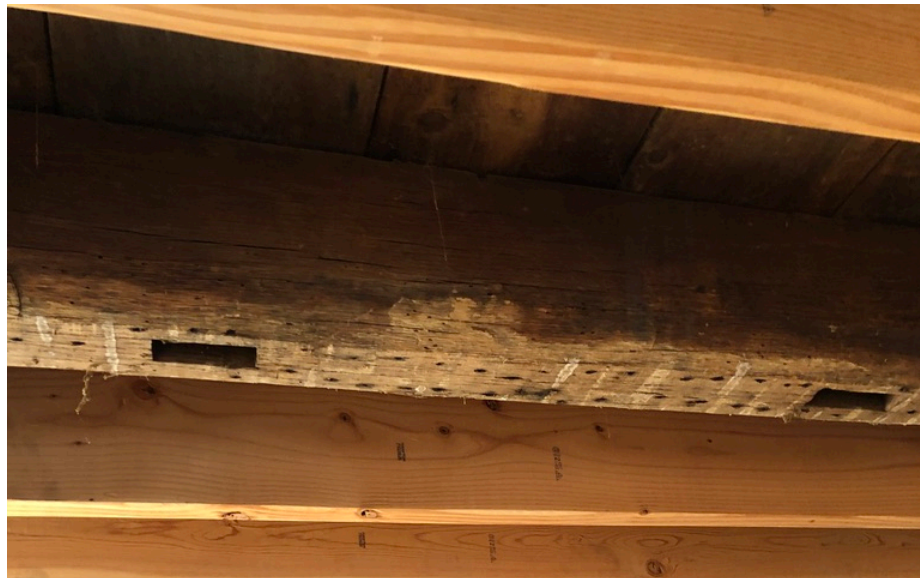
Figure 24. The top image depicts the beam with empty mortises (several of which are obscured by an old strip of lath) outlined in red. The lower image is a close-up of two of the five empty mortises located across the length of the beam. (Source: Francesca Evans, 2022)
