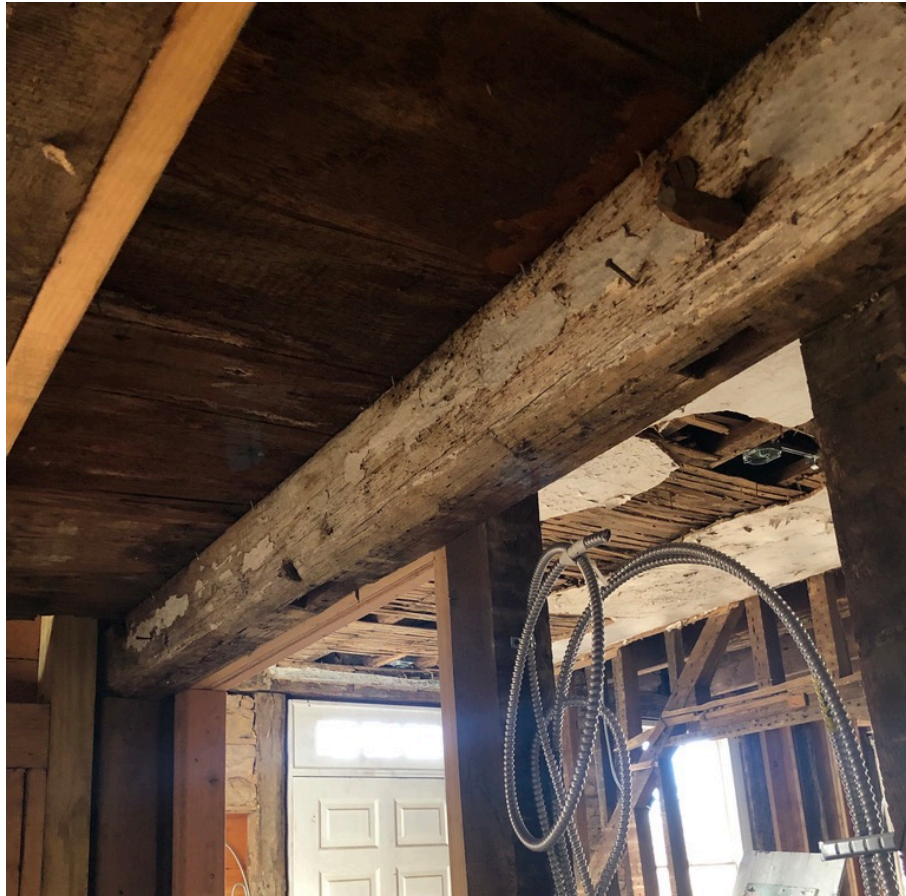
Figure 28. White paint on the northernmost anchor-bent in Phase One. (Source: Francesca Evans, 2022)
