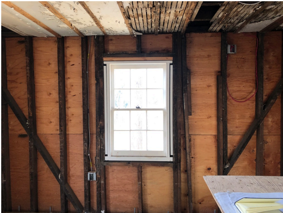
Figure 47. West wall of the Phase Three addition which was built using balloon frame construction. (Source: Francesca Evans, 2022)
