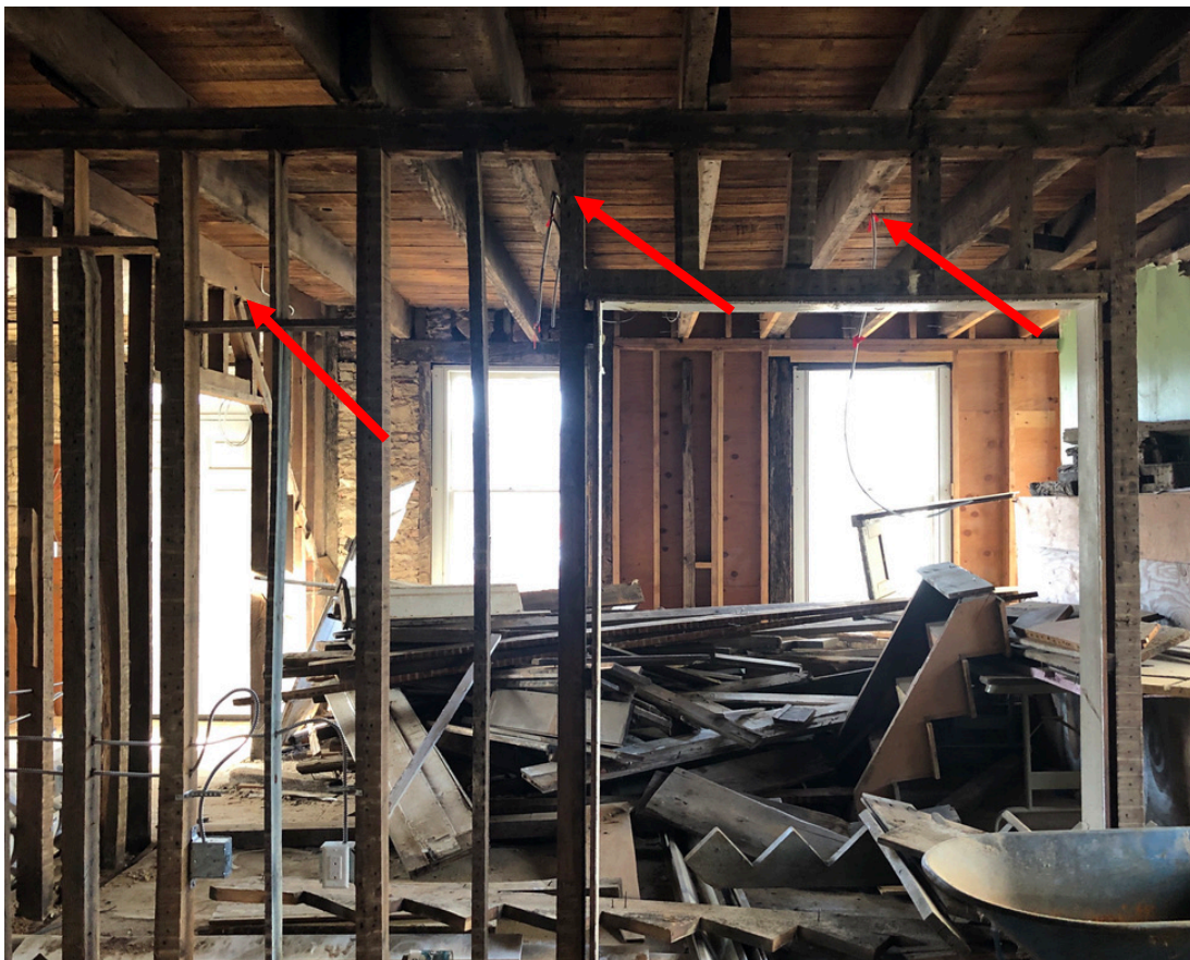
Figure 19. There are only three true anchor-bents (noted by red arrows) in Phase Two, which are connected to a major vertical support in each wall and span the entire width of both parlors. The remaining joists rest atop the beam creating the dividing wall between the two parlors. This dividing wall acts like a summer beam, supporting the joists in each parlor, but lacks the size necessary to be considered a true summer beam as it is supported with the use of studs. (Source: Francesca Evans, 2022)
