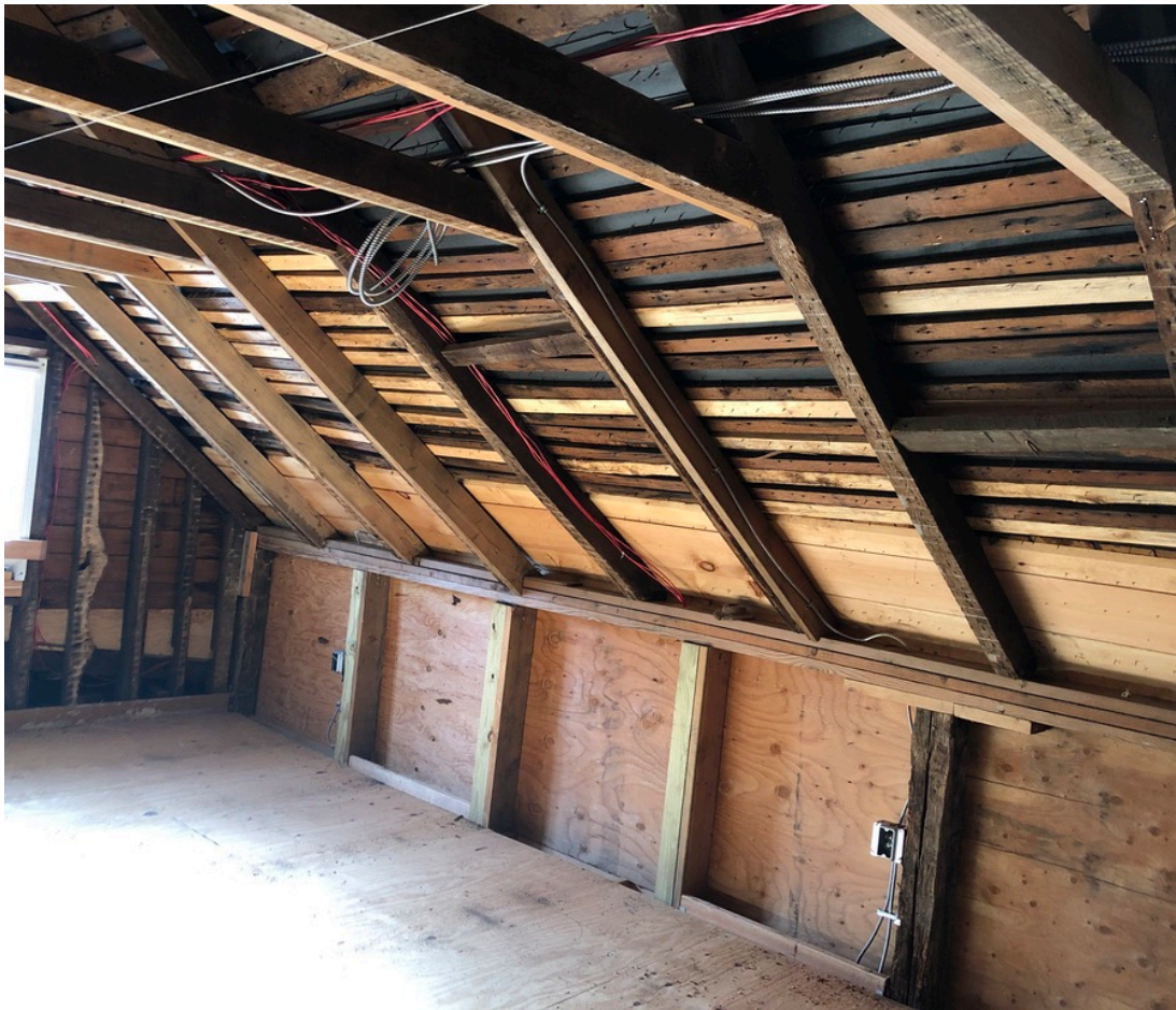
Figure 20. Knee wall extension in the west wall of Phase One. (Source: Francesca Evans, 2022)
