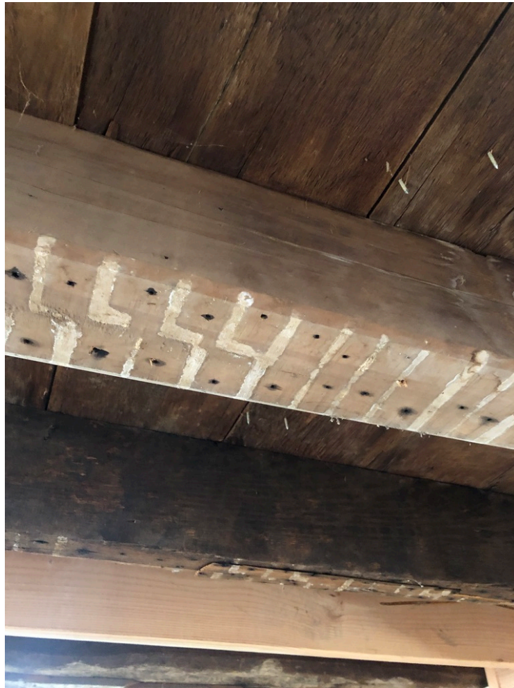
Figure 29. Chamfered edge on one of the planed anchor-bents. (Source: Francesca Evans, 2022)
