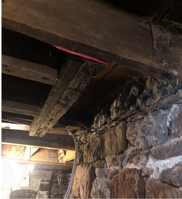
Figure 27. Timber in northeast corner of the cellar under Phase One that may have acted as a header for the stair opening of the original bulkhead. (Source: Francesca Evans, 2022)
