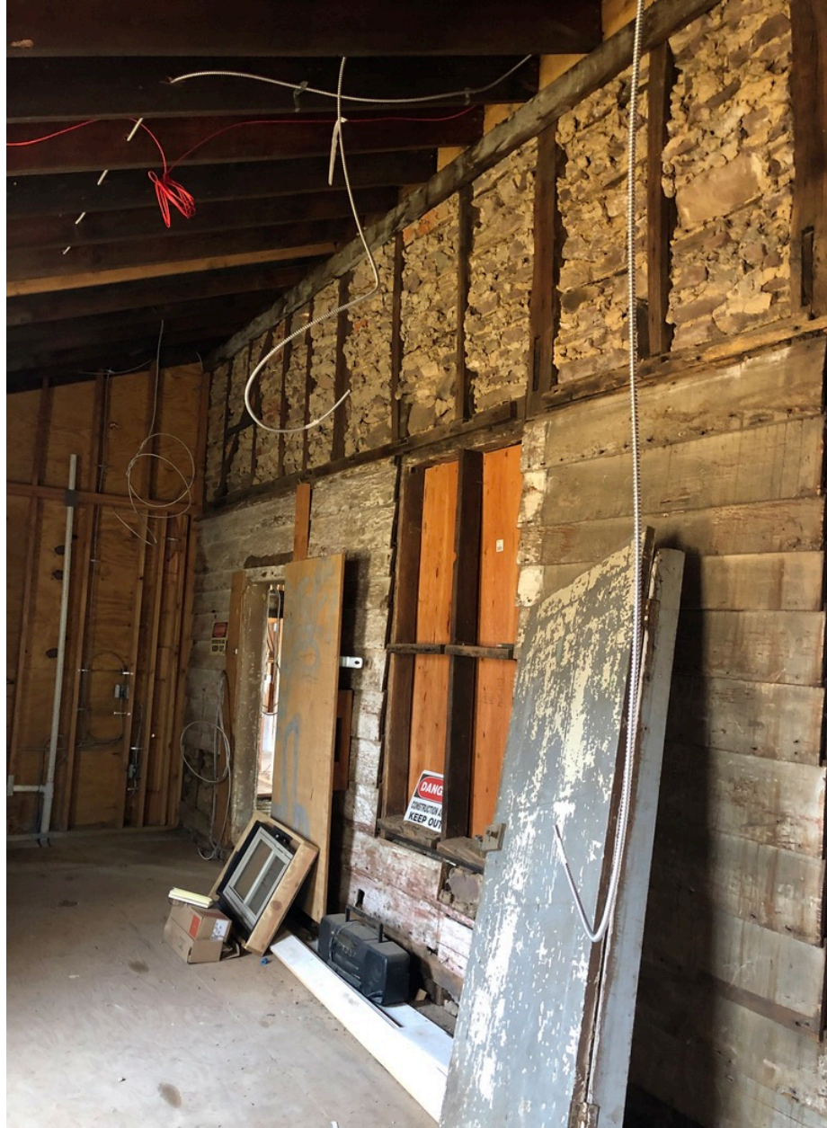
Figure 54. Interior of the Phase Four addition appended to the east of the Phase Two addition. Documentary evidence shows that the original clapboard siding and window were covered over with plaster at some point. (Source: Francesca Evans, 2022)
