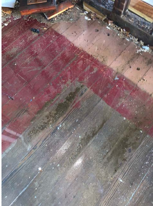
Figure 39. Image of the painted flooring in the east parlor. Note how it is wider than the flooring used in the hall, which is the same flooring that is also found in the west parlor. (Source: Francesca Evans, 2022)
