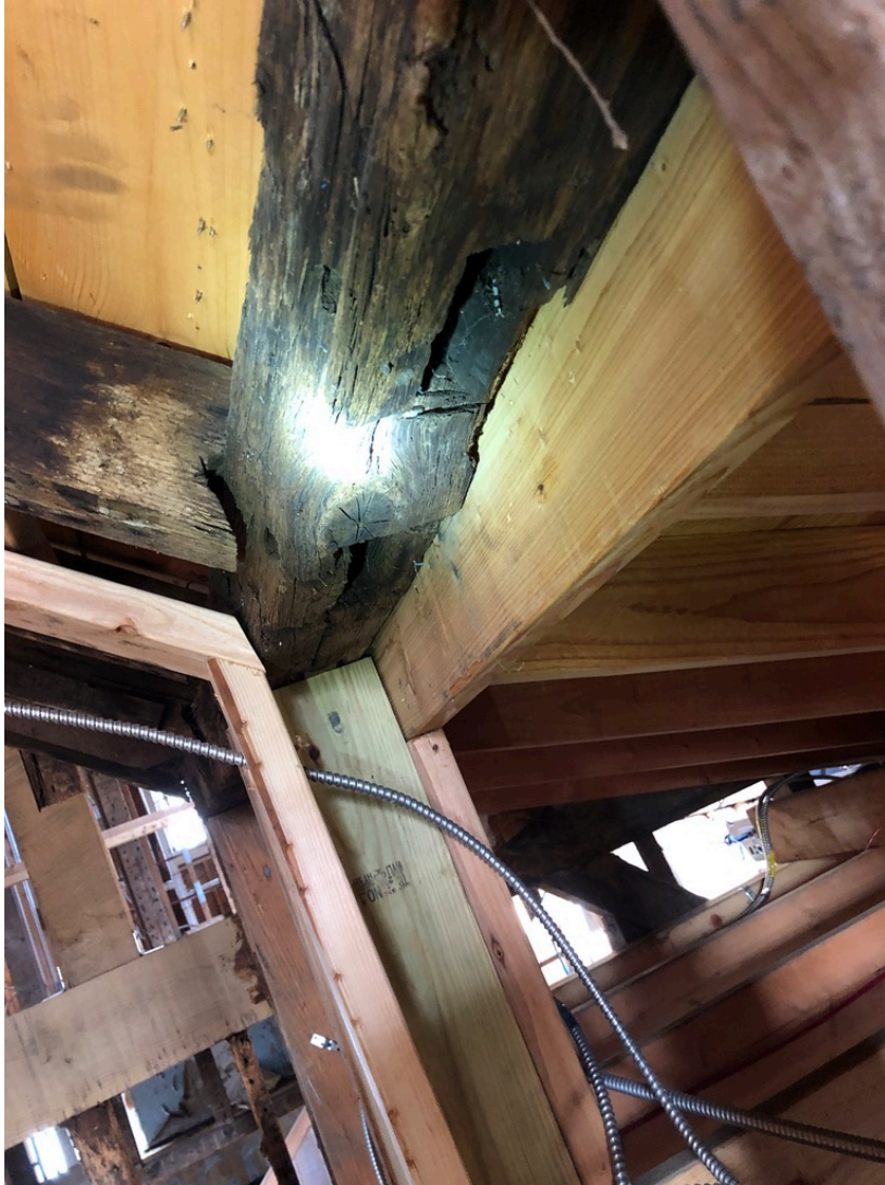
Figure 31. Two empty mortises with peg holes in the top plate of the east wall. (Source: Francesca Evans, 2022)
