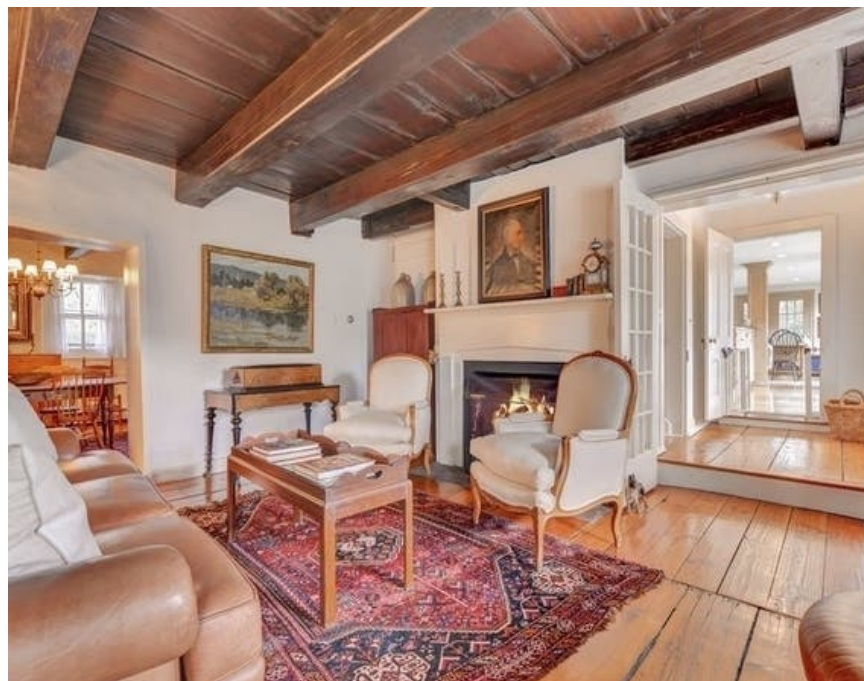
Figure 14. Interior image of the Thomas Van Buskirk House in Saddle River, New Jersey. Note the large, closely spaced anchor-bents running the width of the room and lack of joists in between each bent, compared to the two massive summer beams in Figure 13. (Source: Patch.com)
