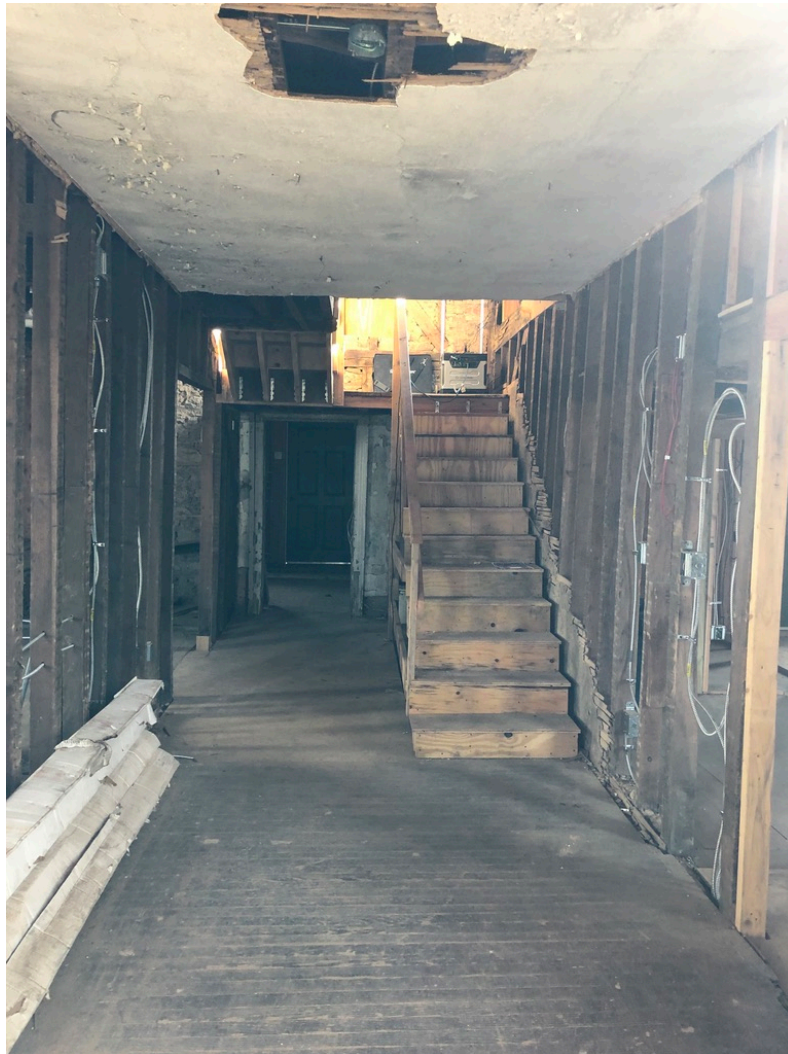
Figure 37. Side hall in the c. 1820 section facing east. The narrow tongue and groove floorboards run north to south in the same direction as the floor joists in the cellar below the hall. When examining the flooring underneath the staircase, it appears as though the original flooring in the hall ran east to west. (Source: Francesca Evans, 2022)
