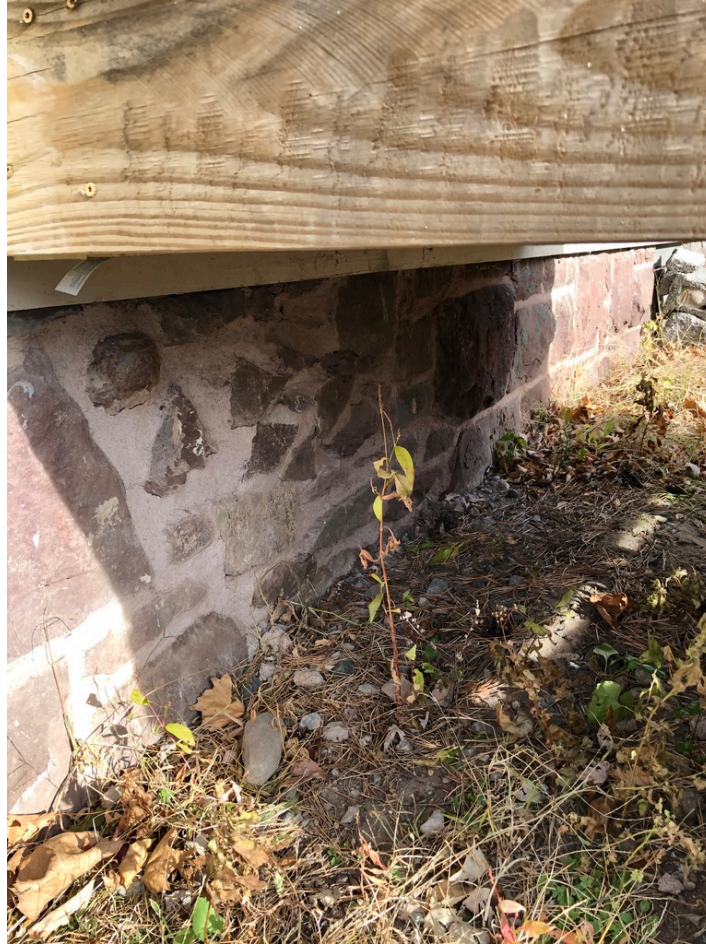
Figure 48. Evidence in the Phase Three foundation of a three-foot wide entry step, most likely added when Phase Three was converted to a gable roof. (Source: Francesca Evans, 2022)
