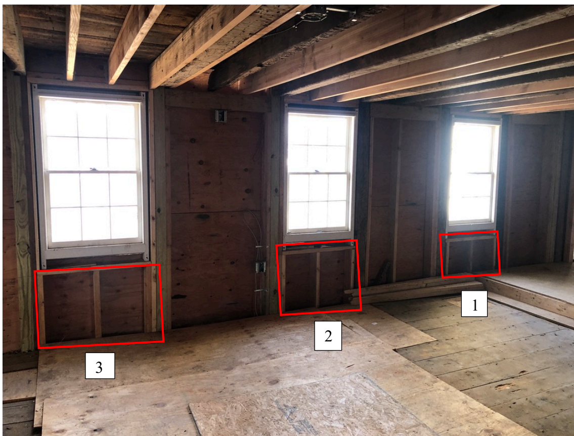
Figure 23. Facing West: Anchor-bents and additional structural supports from the stabilization of the building. Prior to the rehabilitation, nogging was found in bays one and two while none was found in bay three, leading the National Register nomination authors to suggest that bay three contained the original entry. (Source: Francesca Evans, 2022)
