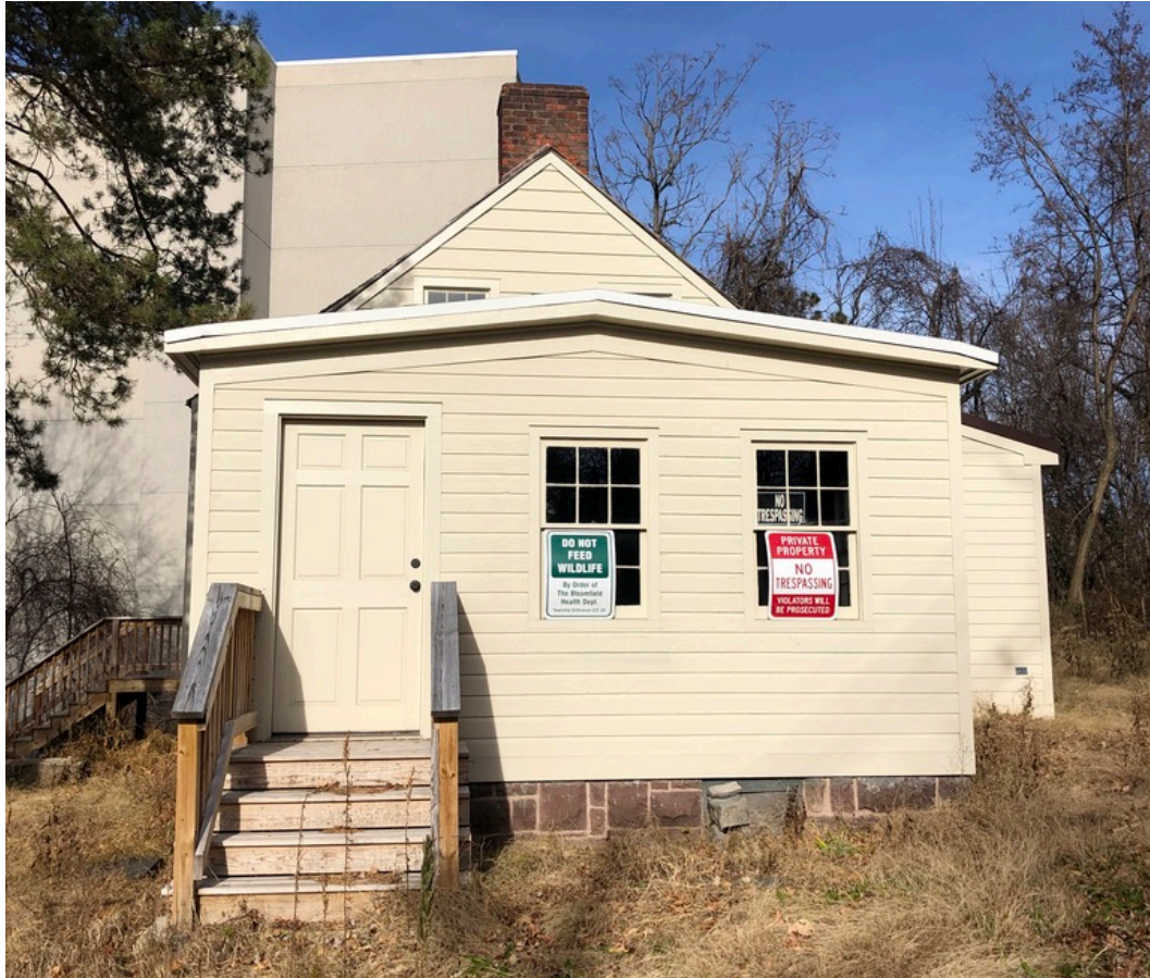
Figure 45. South façade of the Phase Three addition. Note the difference in appearance from Phases One and Two, especially the one-story height, low roof pitch, foundation appearance, and German drop siding. (Source: Francesca Evans, 2022)
