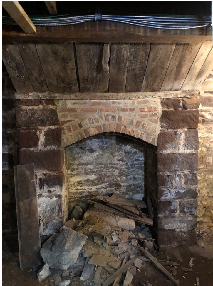
Figure 35. Lower supports for the fireplace in the west parlor. Note the brick segmental arch which was added later. (Source: Francesca Evans, 2022)
