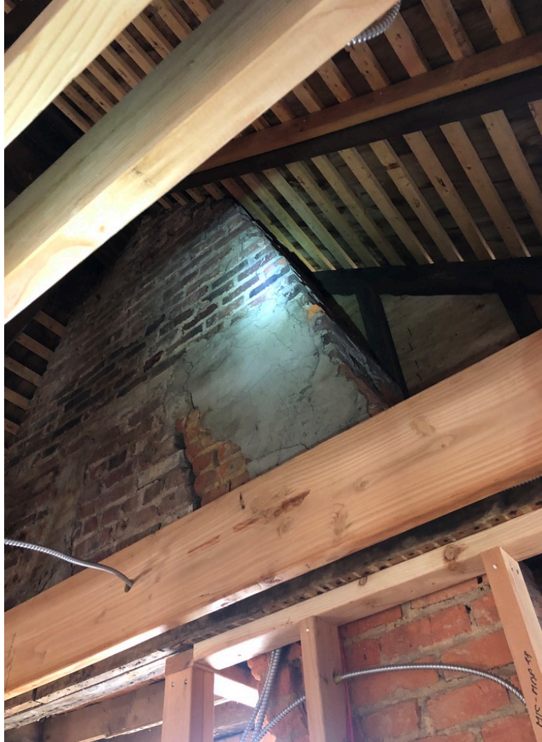
Figure 40. Evidence of repairs made to the double chimney. (Source: Francesca Evans, 2022)
