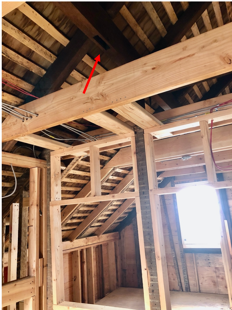
Figure 42. One of three empty mortises in the purlin on the west side of the roof. The post, reinforced on either side by new lumber, is mortised into the purlin, providing evidence that similar posts would have been in the three empty mortises, effectively dividing the half-story space. (Source: Francesca Evans, 2022)
