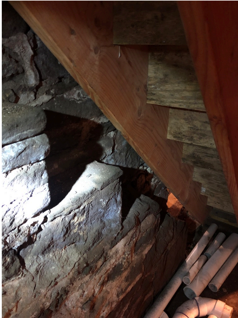
Figure 36. This stepped ledge in the southern wall of the Phase Two cellar indicates where an earlier staircase was located. (Source: Francesca Evans, 2022)
