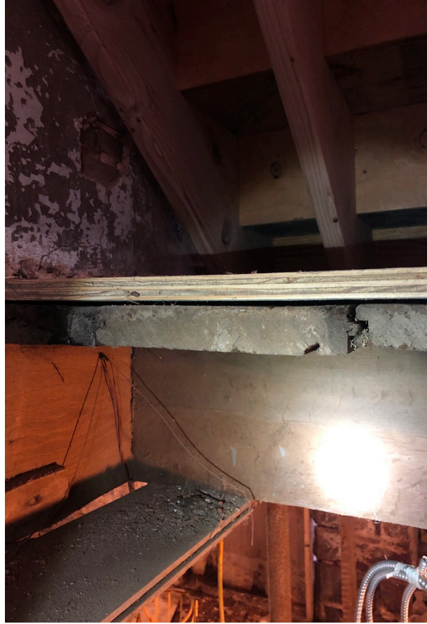
Figure 38. Image of the flooring that remains underneath the staircase. Note the north-south direction of the joists which run throughout the side hall and the east-west direction of the flooring. This flooring runs underneath the current flooring in the stair hall and is much wider as seen in Figure 37. (Source: Francesca Evans, 2022)
