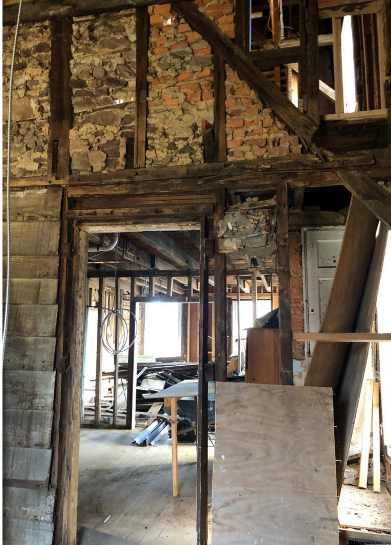
Figure 56. Doorway leading into the Phase Two addition from the Phase Four addition. This doorway was once a window, prior to the construction of the Phase Four addition. A floor plan in the 1982 cultural resources survey shows no opening in this location, while the 2015 National Register nomination does show an opening here (although there is no indication that it is a doorway). It is unclear when the window was converted into a doorway—it could have been before the wall was plastered over or sometime after the cultural resources survey was completed in 1982. (Source: Francesca Evans, 2022)
