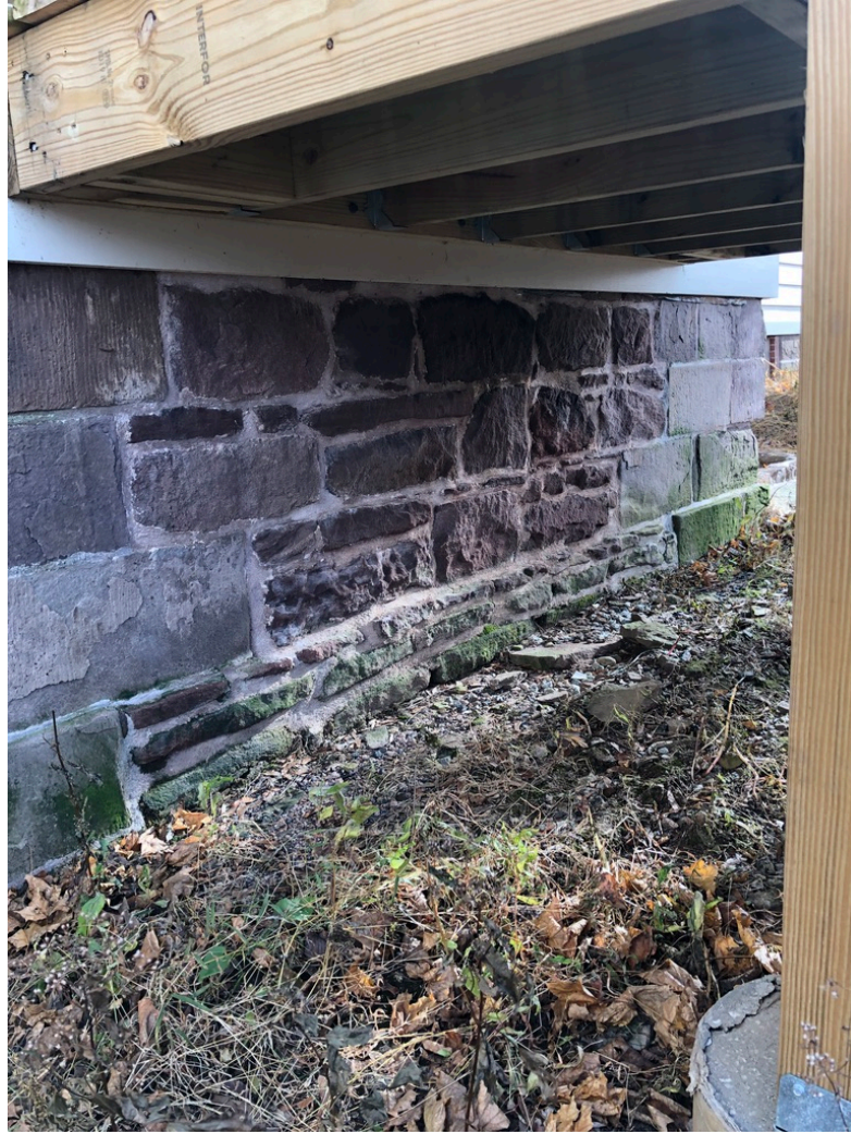
Figure 34. Evidence in the foundation of the location and size of the original front step when this section of the house was constructed. (Source: Francesca Evans, 2022)
