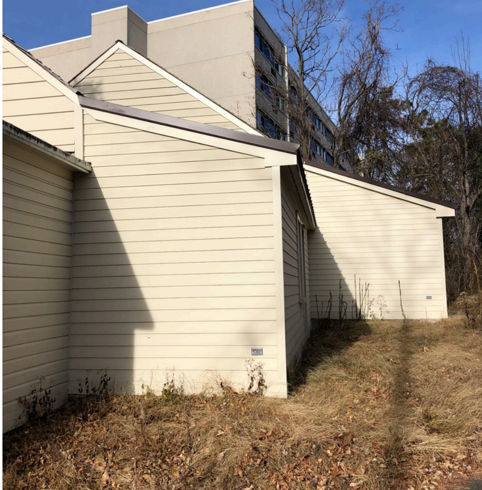
Figure 52. Phase Four additions. Note the difference in siding from Phase Three and the narrower clapboards used than those seen on Phases One and Two. (Source: Francesca Evans, 2022)
