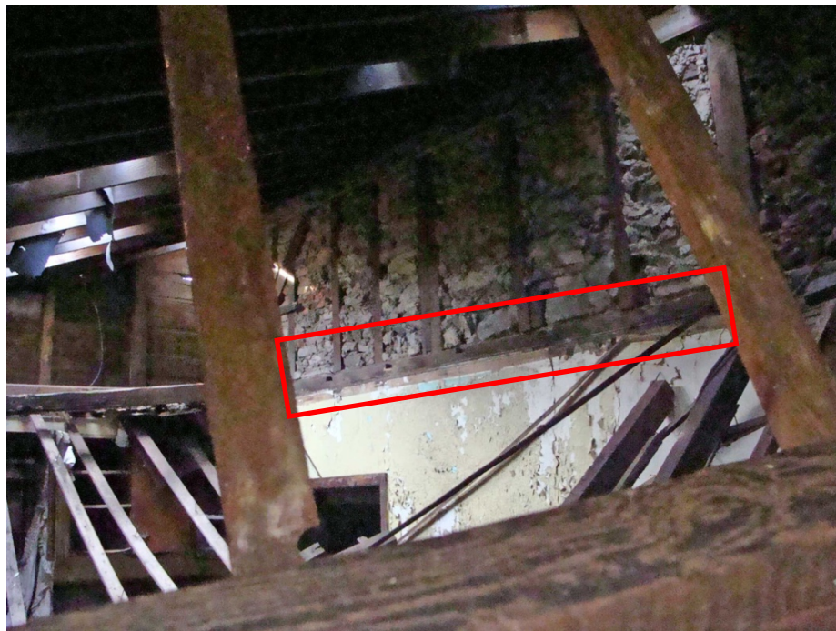
Figure 55. Image taken prior to any stabilization or rehabilitation efforts. Note the plastered wall, pockets in the ledger board (in red), and extant ceiling joists in place (in the far left of the photograph) and those resting on the wall. (Source: Rich Rockwell)
