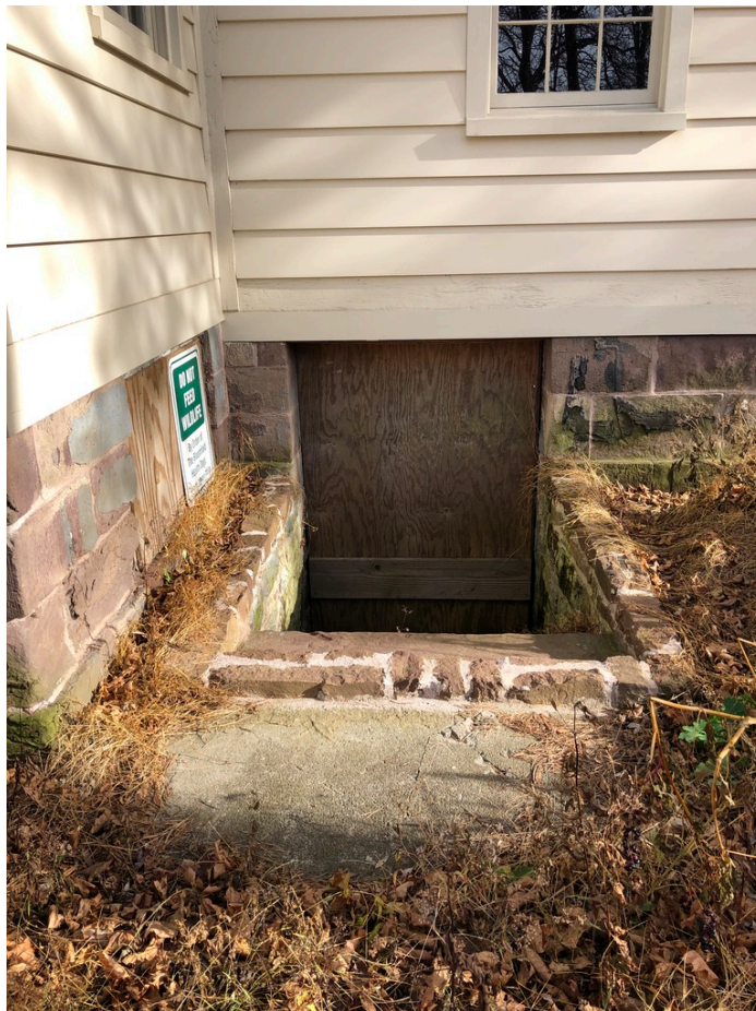
Figure 26. Bulkhead leading to the cellar of the original dwelling located in the first bay of the west façade. Note how it is unaligned with the first story window. (Source: Francesca Evans, 2022)
