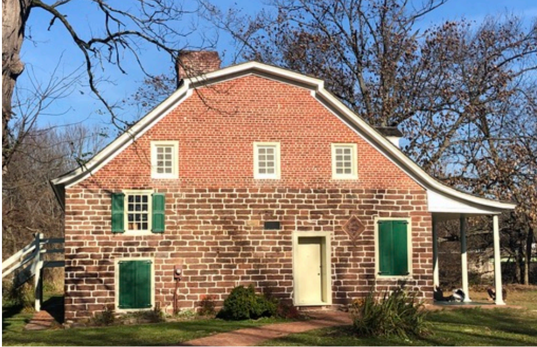
Figure 12. The roof of the Ackerman-Zabriskie-Steuben House in River Edge, New Jersey is representative of the typical gambrel roof form associated with the Dutch-American house type. (Source: Francesca Evans, 2020)
