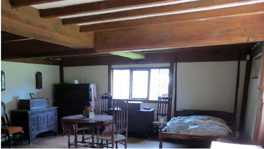
Figure 13. Interior image of the Captain John Whipple House in Ipswich, Massachusetts. Note the two summer beams intersecting in the middle of the room and the smaller joists that run from front to rear of the house perpendicular to the summer beam. (Source: Historic Ipswich)
