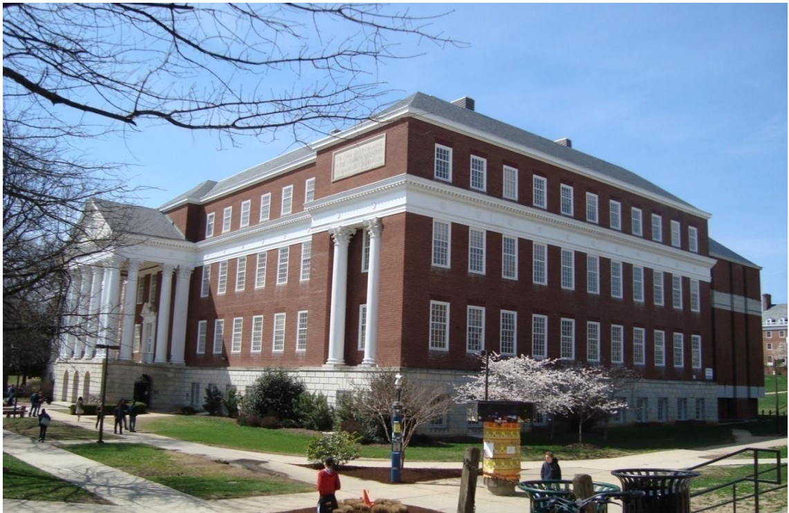
Fig. 32. McKeldin Library, University of Maryland. Existing condition, original building with addition on the back. Digital Photo by Zasha N. Guzmán Torres, March 2, 2009.
