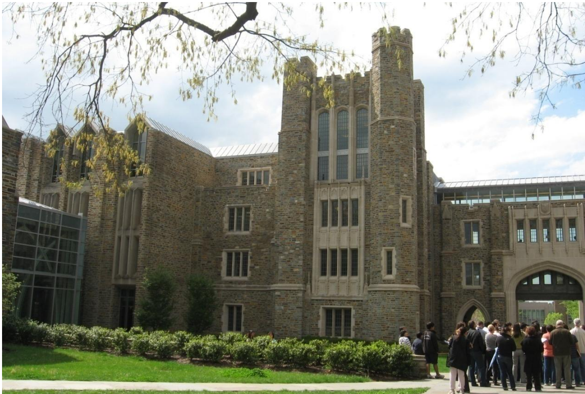
Fig. 4. William R. Perkin Library, Duke University, South Side. First addition on the right, and second addition on the lower left. Digital photo by Cindy Frank, April 6, 2009.
