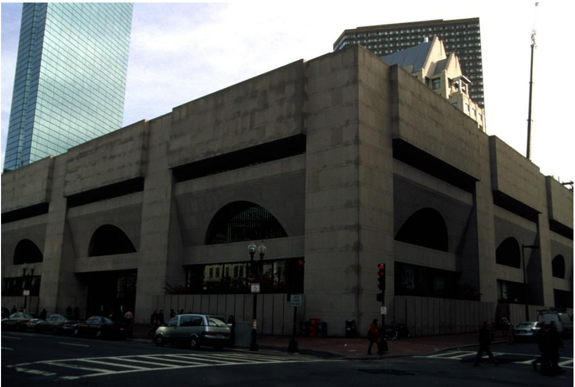
Fig. 20. Boston Public Library Addition. View of corner with Hancock Bldg. Image property of R. L. Vann.
