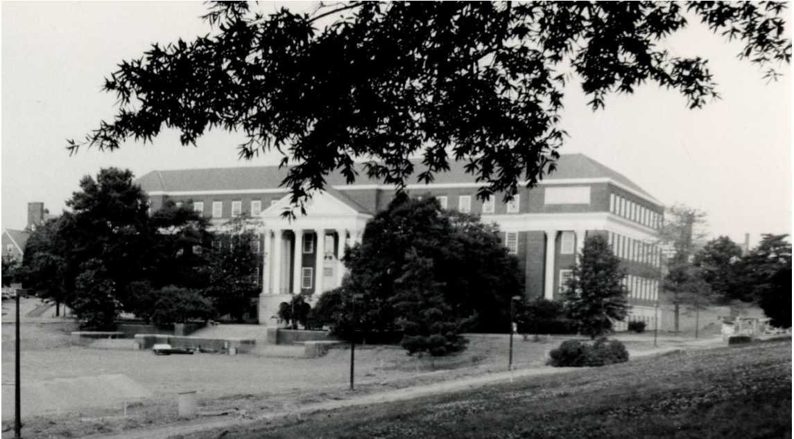
Fig. 29. McKeldin Library, University of Maryland. Original Building. Image by University of Maryland.
