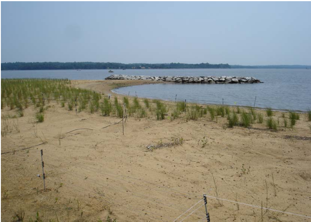
Figure 15. Restored shoreline at Trent Hall Farm beach with breakwater addition providing more openings for terrapins to reach the beach and nest. (Team Saving Testudo Research Collection)
