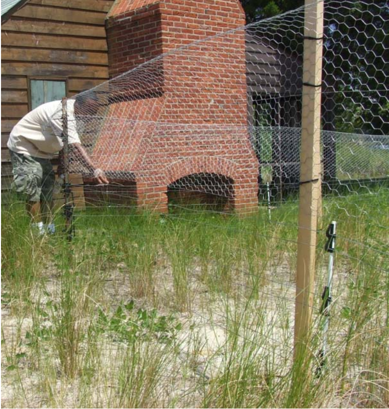
Figure 22. Addition of chicken wire mesh to fence design at Jefferson Patterson Park and Museum, 2008. (Team Saving Testudo Research Collection)
