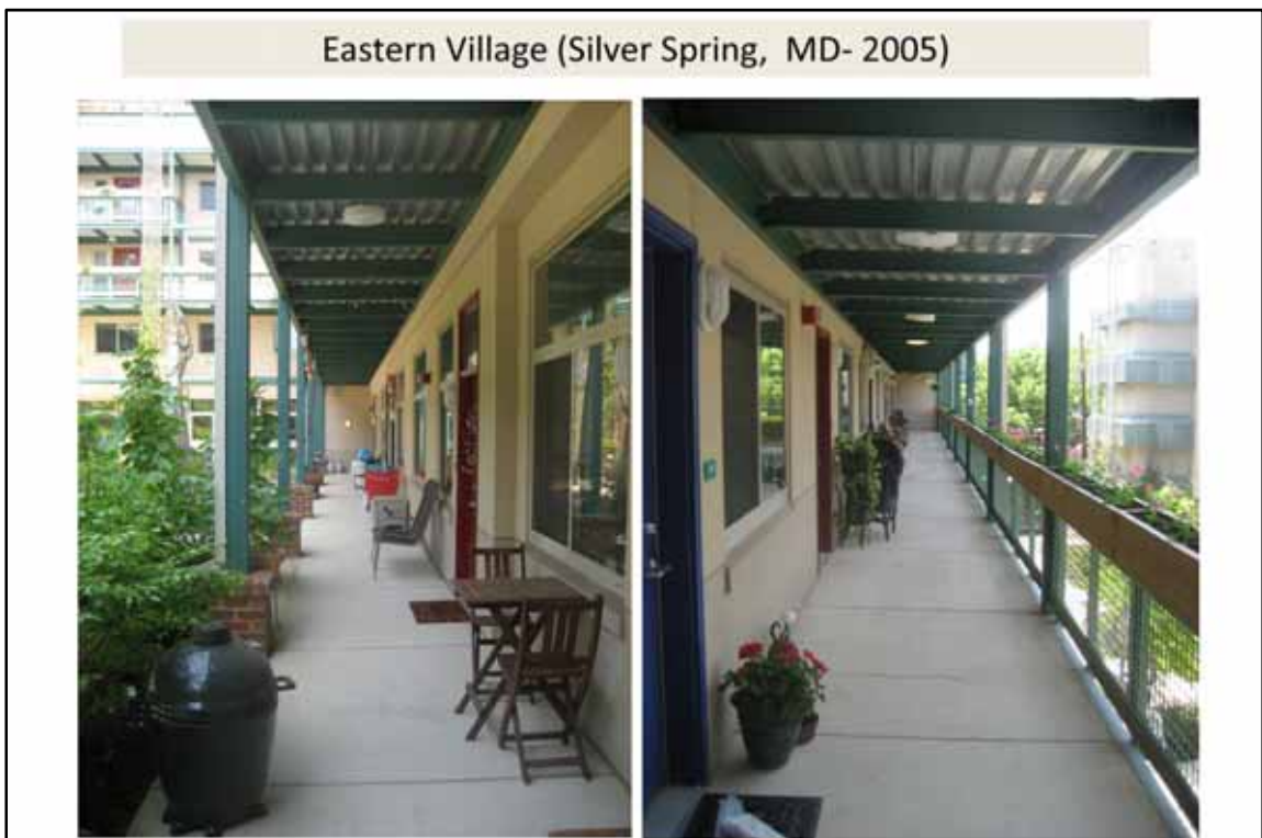
Figure 49: Eastern Village Exterior Corridors.
