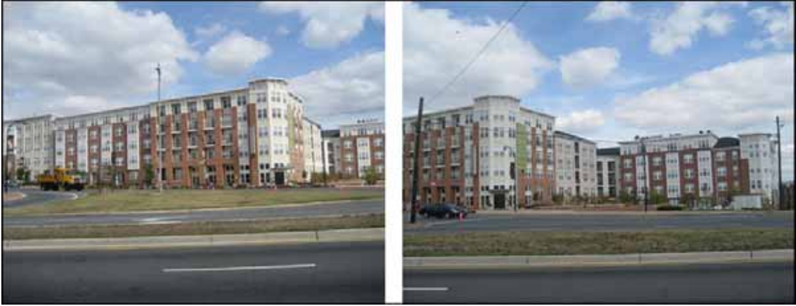
Figure 30: The Montgomery Apartments, Wheaton, MD.
