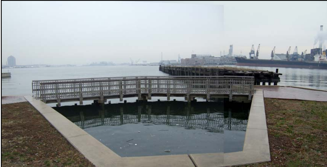
Figure 17 Existing Walkway and Pier
