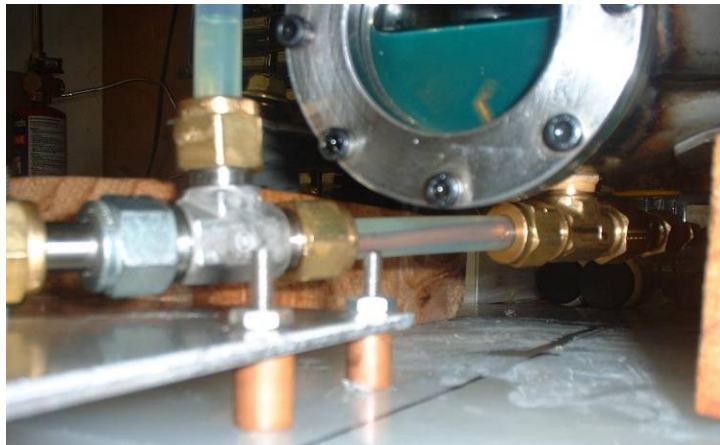
Figure 47: Sample Collection Pipe through the Sight Tube at the bottom of the Compressor
