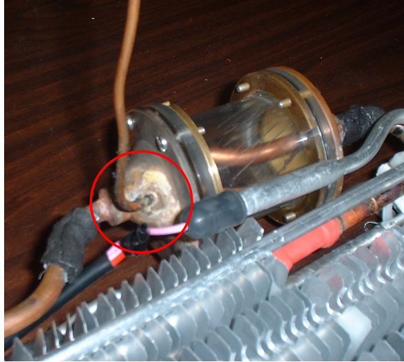
Figure 49: Sample Pipe in Accumulator (rear view)
