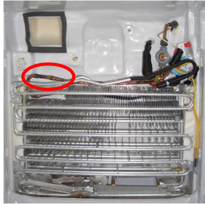
Figure 86: Accumulator Removal and Pipe Replacement
