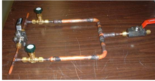
Figure 52: Oil Charging "U" Tube
