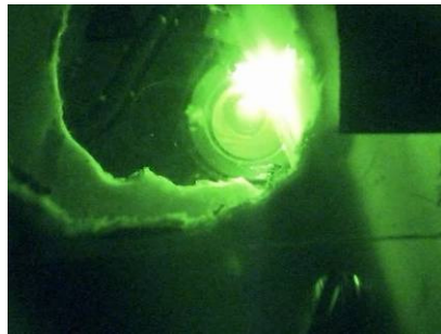
Figure 22: Camera View of the Accumulator Outlet with LED Lights
