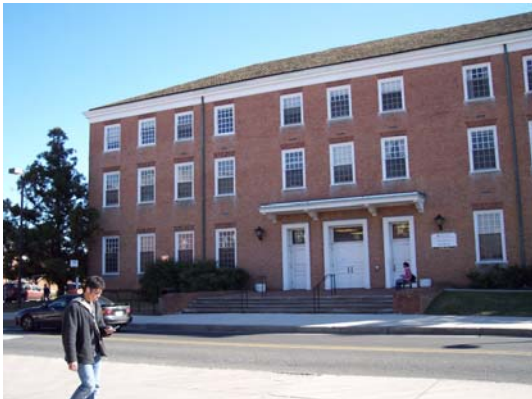
Fig. 13: Benjamin Building across the street (©2006 C. M. Newburn)
