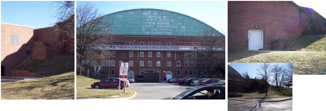
Fig. 7: Stair from east end of terrace; North facade; Walkway down from terrace (©2006 C. M. Newburn)
