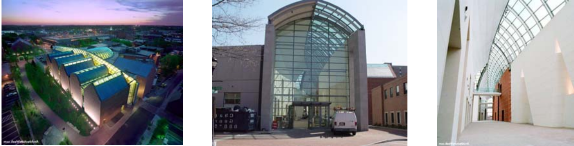
Fig. 57: Aerial, exterior, and entrance ( www.architectureweek.com )
