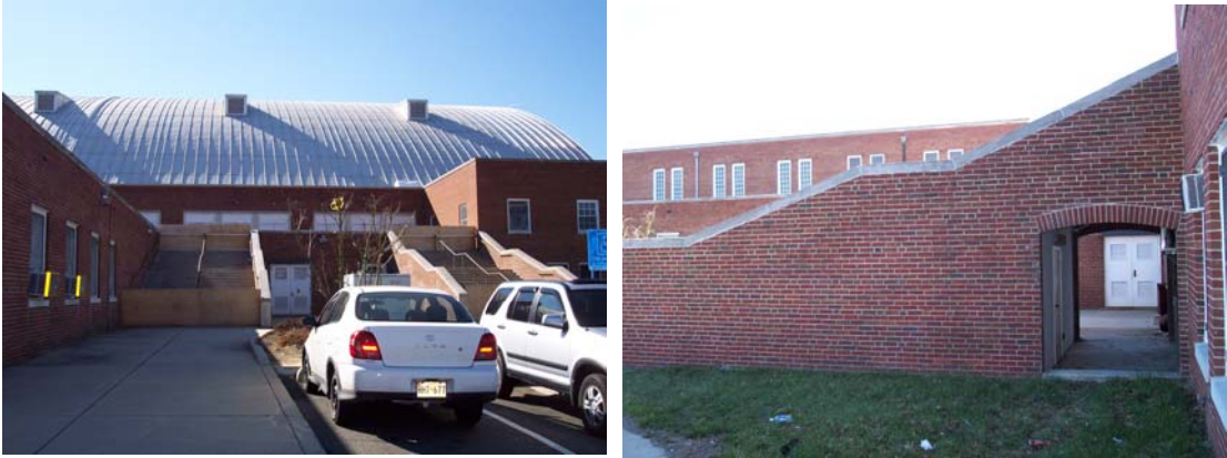
Fig. 17: Exit stairs (now blocked); Exit stairs (Pool House behind) (©2006 C. M. Newburn)
