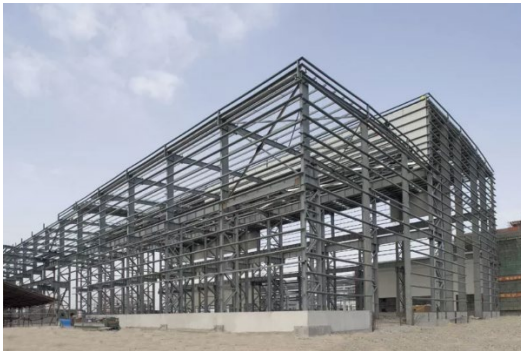
Figure 21: China Prefab Industrial Steel Buildings. (Source: Hangzhou FAMOUS Steel Engineering Co., Ltd.)
