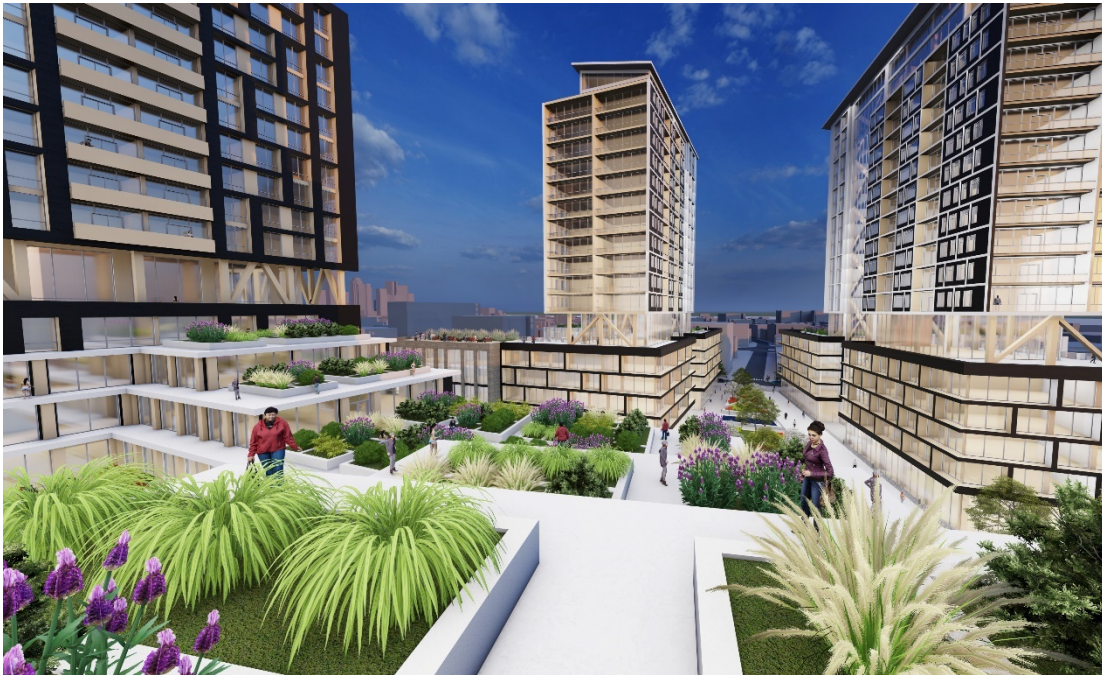
Figure 46: One of the Various Green roofs at Cayler Point. (Source: Author)
