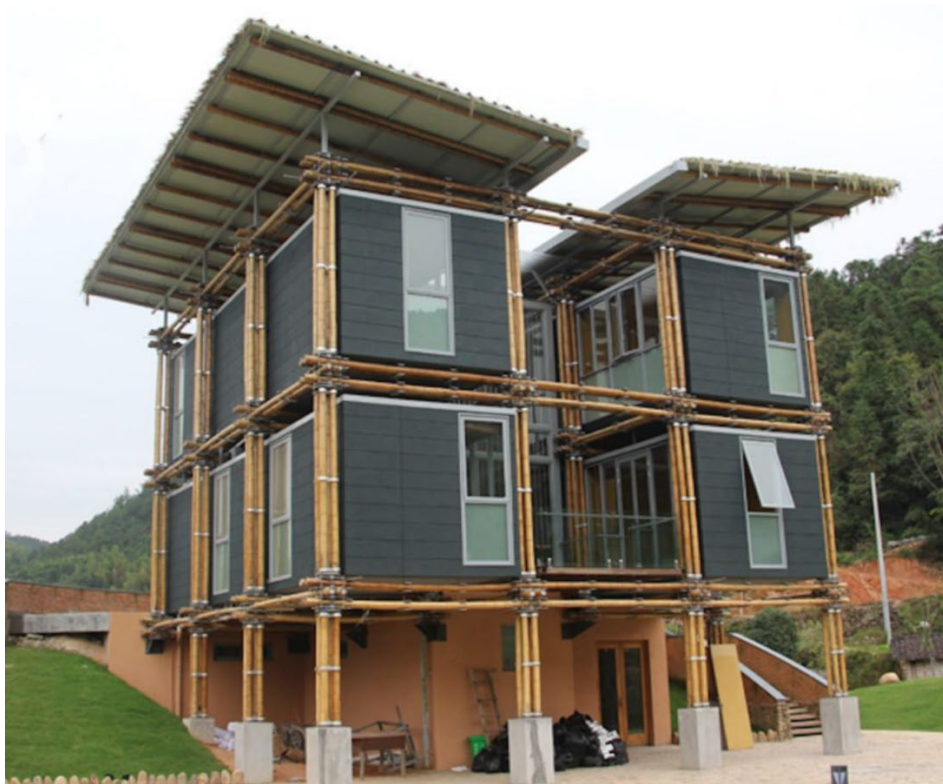
Figure 20: This experimental bamboo home is helping to set the pace for sustainable growth in China. Milan-based Studio Cardenas designed Energy Efficient Bamboo House, a home with a minimal carbon footprint and Feng Shui-inspired construction. Located in the Longuan International Bamboo Commune in Zhejiang, the energy-saving adobe uses locally available natural materials to create a cost-effective building that saves substantially on energy use. (Source: Lucy Wang)
