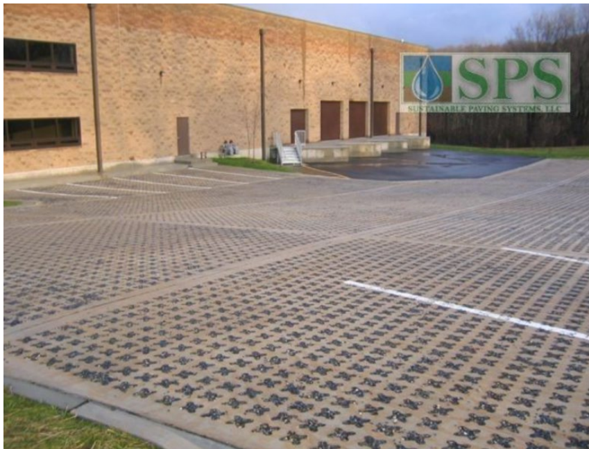
Figure 19: Grasscrete stone filled system at Plum Way II Commercial Building. (Source: Sustainable Paving Systems, LLC)
