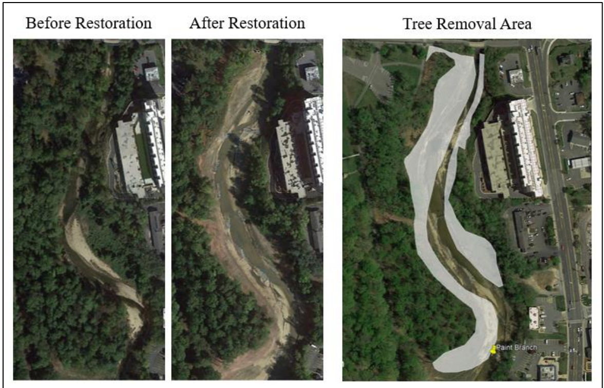
Figure 2: Tree removal at Paint Branch during stream restoration. Before (2012) After (2014)
