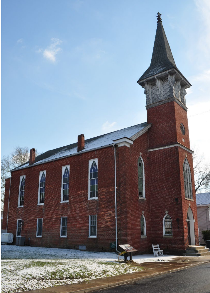
FIGURE 3.1: Asbury United Methodist Church. This church has its origins in African-American involvement in local Methodism in the late eighteenth century and was organized in the antebellum period as a separate congregation. It remained within the Methodist Episcopal Church until that denomination's merger in the twentieth century, which created the United Methodist Church. The congregation purchased this lot in 1849 and the current building dates to 1876. The steeple was added later.
