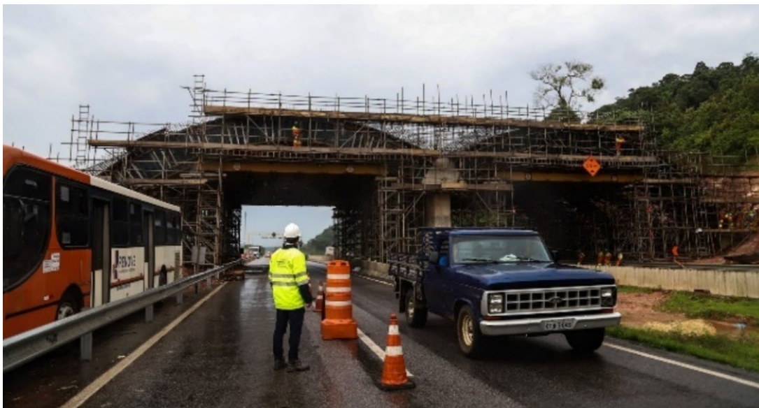
Figure 6. Vehicle view of wildlife crossing under construction (James Dietz)
