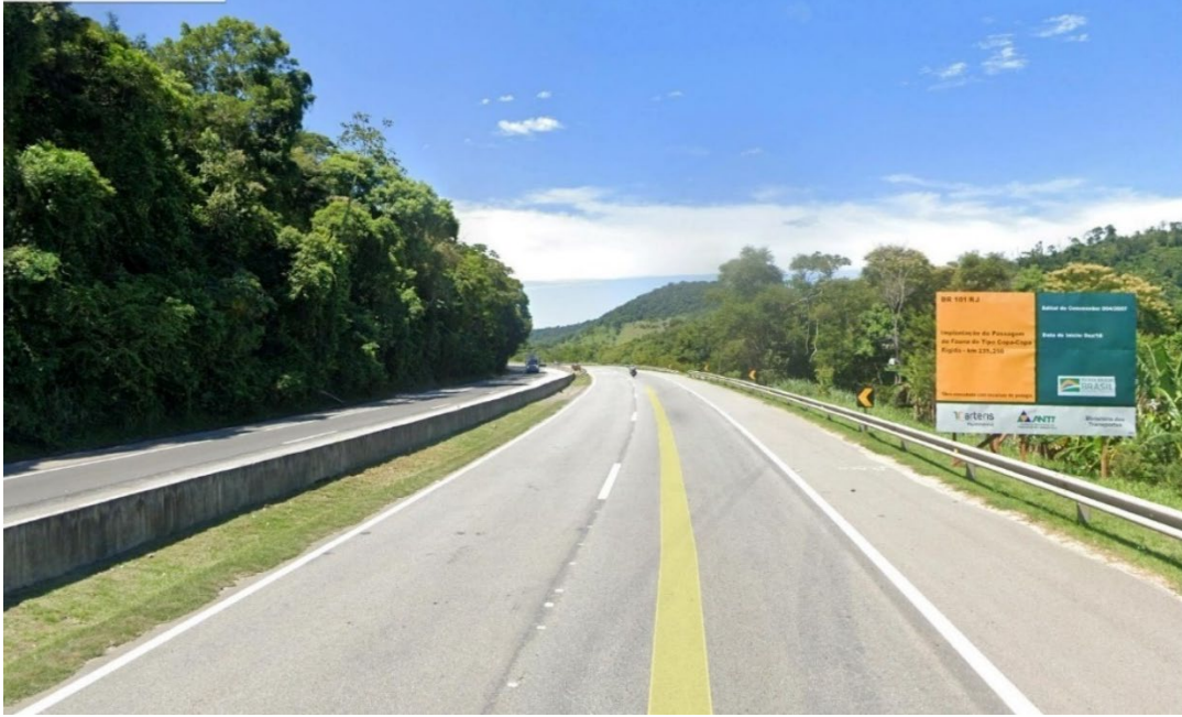
Figure 10. Eastern view of Site 3 (Google Earth)
