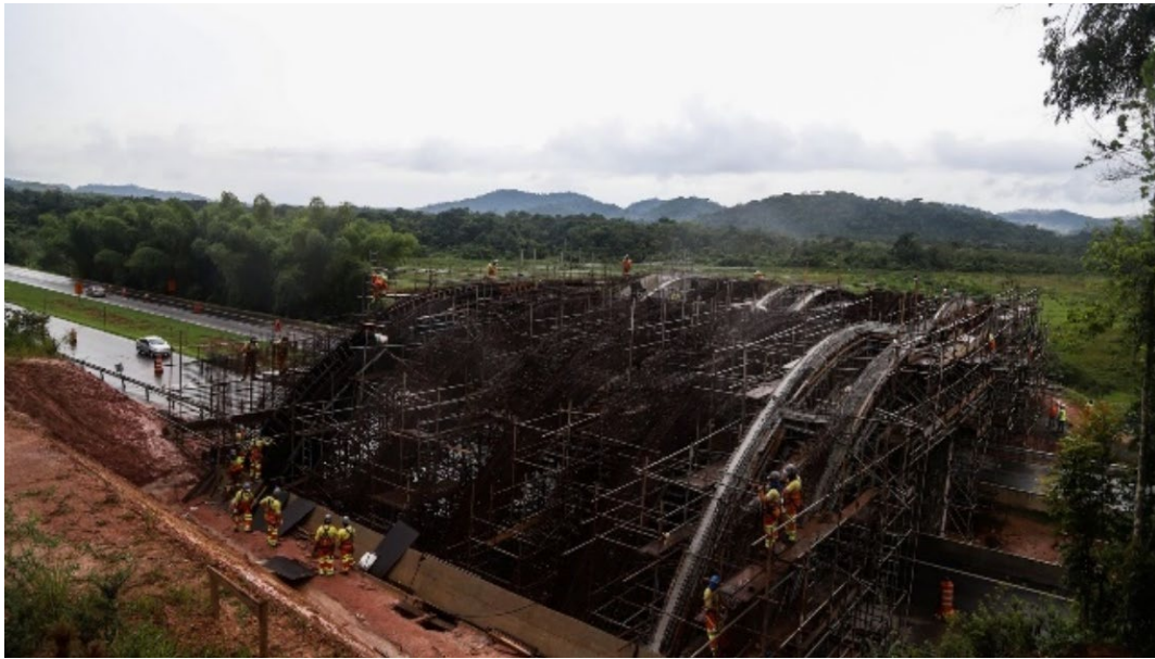
Figure 7. Bird's eye view of wildlife crossing under construction (Gorman, 2020)
