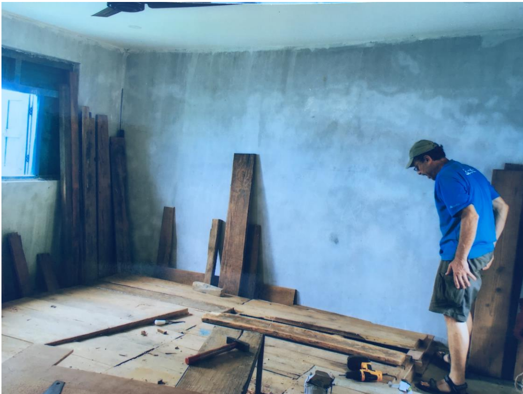
Figure 8: Saipal - French volunteer building classroom floor
