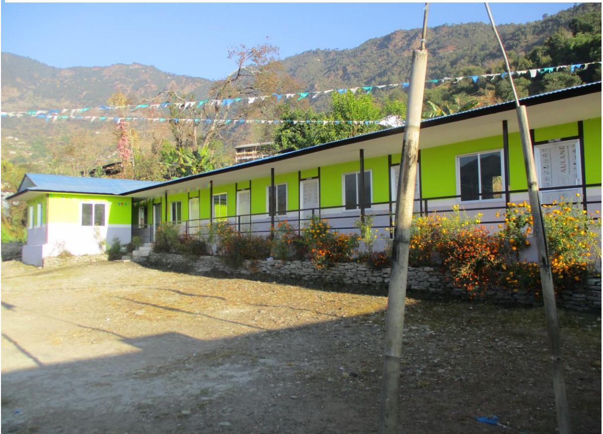
Figure 5: Kabru - Rebuilt School Building
