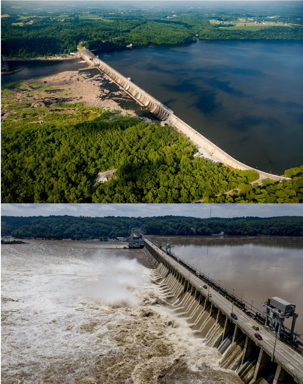
Figure 1.2. Aerial photos of the Conowingo Hydroelectric Dam and reservoir during typical (top, Photo Credit: Will Parson, Chesapeake Bay Program) and high (bottom, Photo Credit: Cecil Whig) river discharge conditions.
