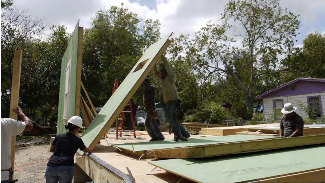
Figure 5.5: Panelized Wall System of Rapido's Core Module Source: Omar Hakeem Lecture
