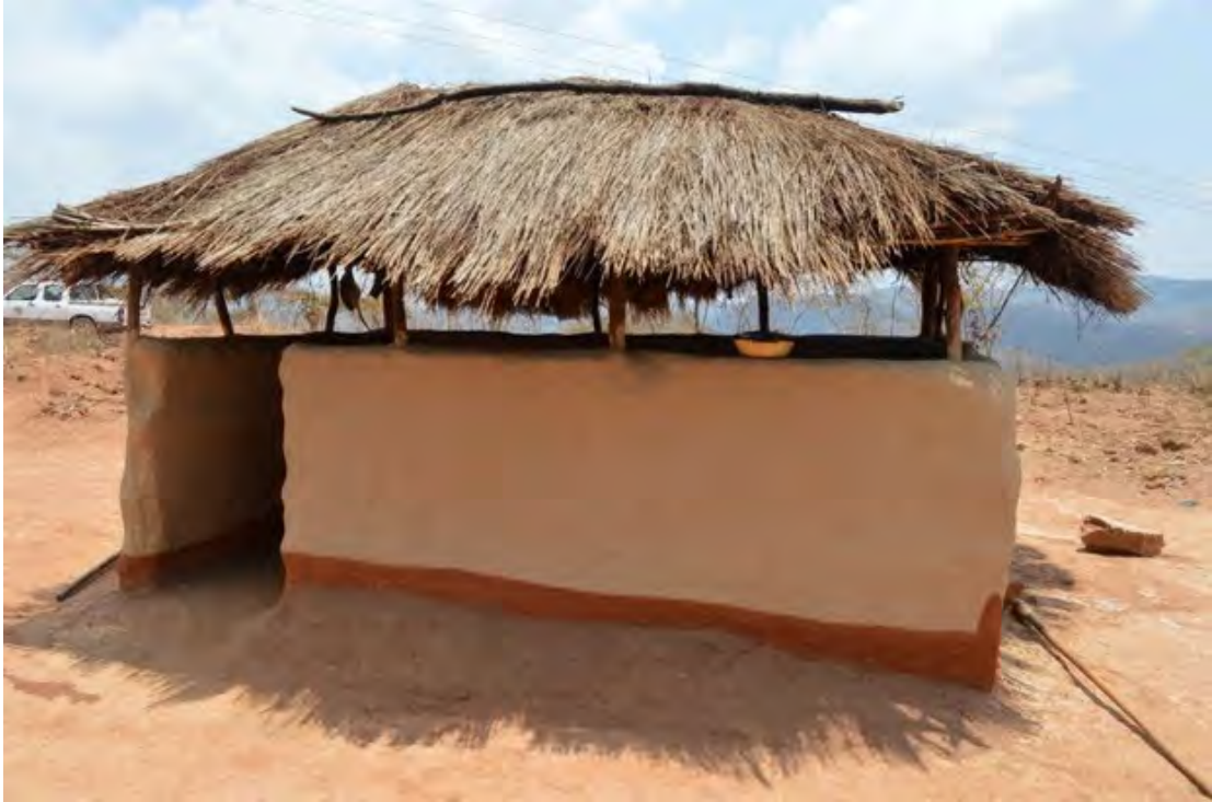
Figure 6.12: Open-Air Construction in DRC Source: Architectural Review
