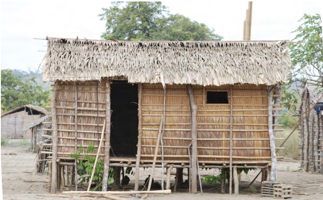
Figure 6.13: Above-Ground Construction in DRC Source: Architectural Review
