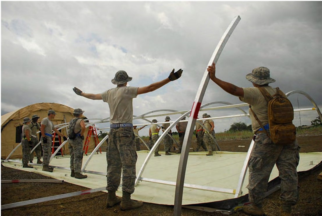
Figure 6.2: Structure Assembly of MMU Source: United States Africa Command
