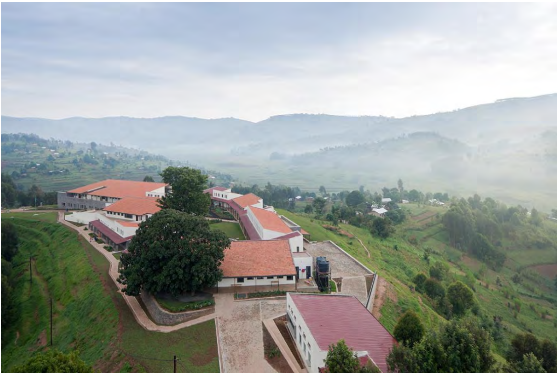
Figure 8.1: The Butaro District Hospital on a Terraced Hillside
