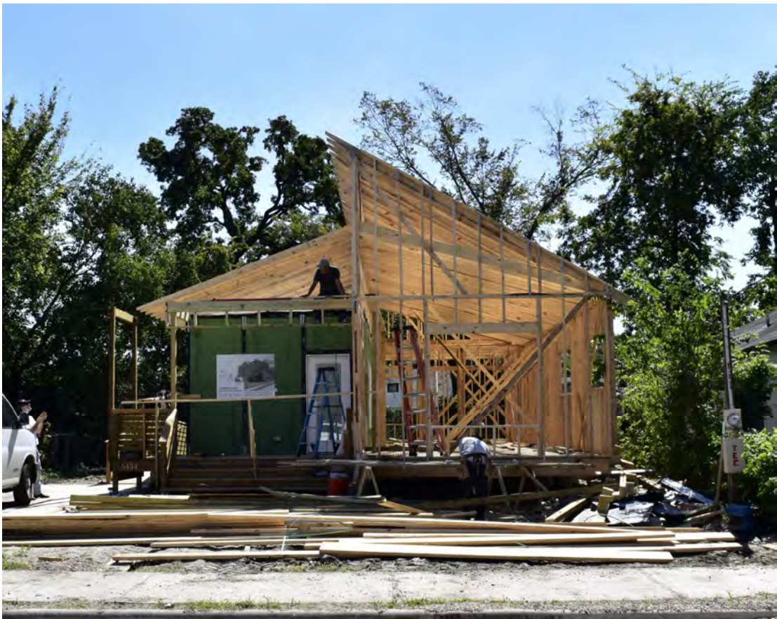
Figure 5.6: Wood Frame Addition onto Core Module Source: Omar Hakeem Lecture
