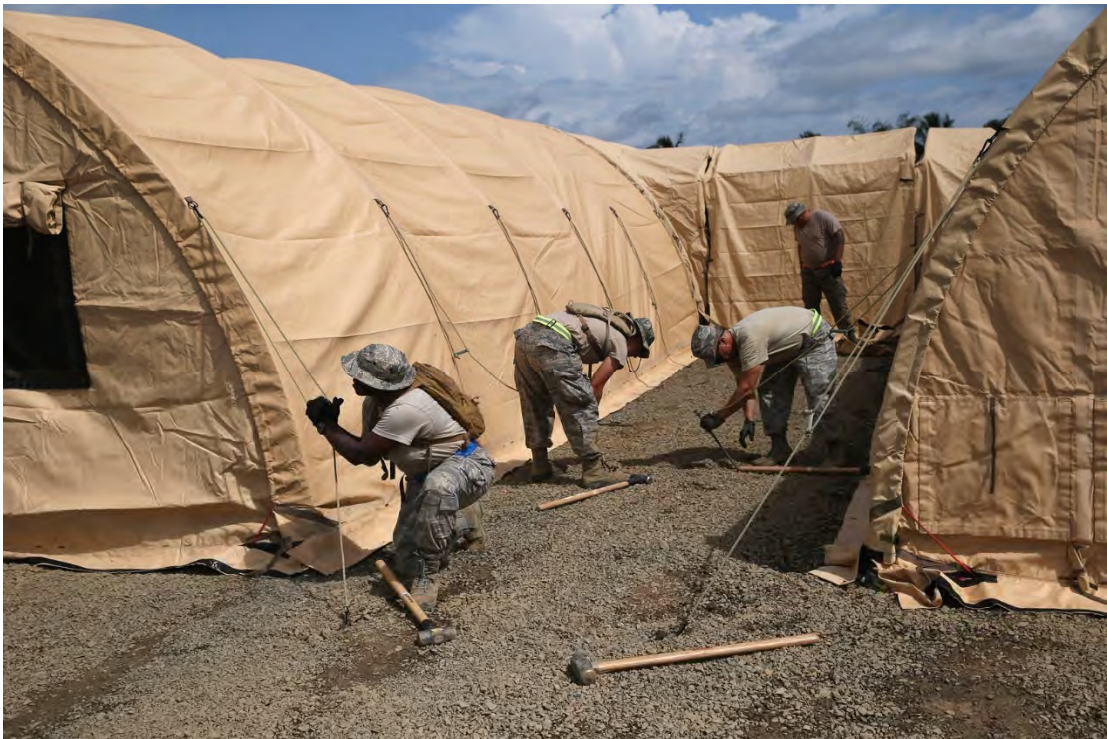
Figure 6.3: Military Tying Down Tarp Over MMU Structure Source: Designboom
