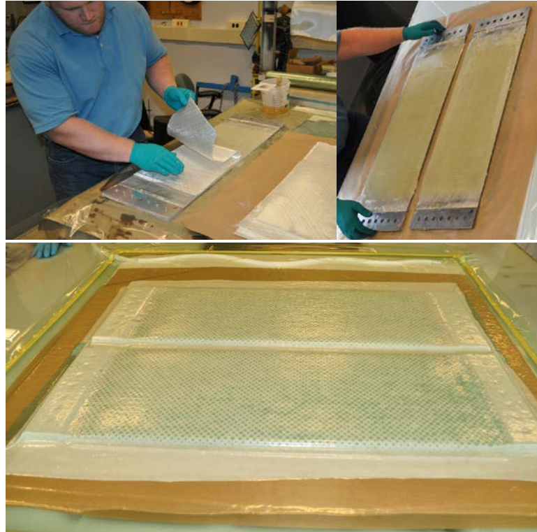
Figure 5-6 Large scale CCT lamination procedure. Clockwise from the upper left the plies are placed and wet-out with resin. Once fully impregnated with resin the laminate stack is applied and vacuum consolidates the stack.
