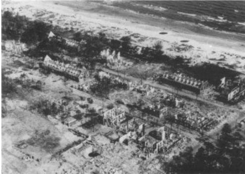
The employee settlement was badly damaged during the British air raid of August 17/18. Courtesy DM
