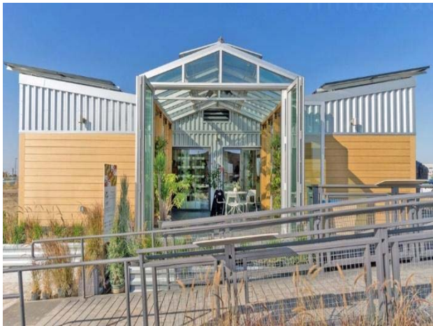
Figure 8: Front view of sd2017 reACT with opened Greencourt, the center of collected passive heat ( sd2017 Team Maryland reACT , 2017)
