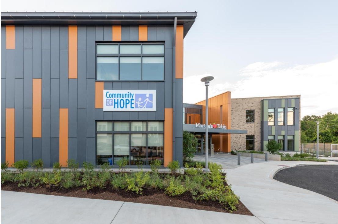
Figure 17, Image of Martha's Table Building Exterior
