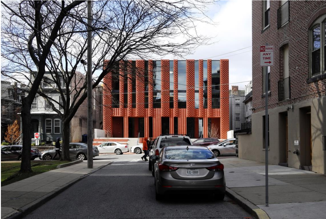
Figure 30, Image of The Center for Jewish Life Building Exterior
