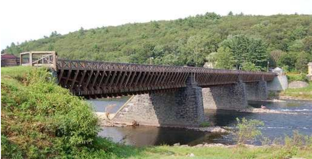
Figure 3. Roebing's Delaware Aqueduct Source: Derek Ramsey, Wikimedia Commons, accessed March 16, 2018, https://commons.wikimedia.org/wiki/File:Roebing%27s_Delaware_Aqueduct_Side_View_3000px.jpg
