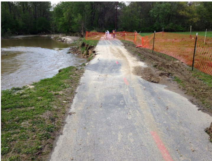
Streambank erosion can also impact public infrastructure like this biking and walking path.
