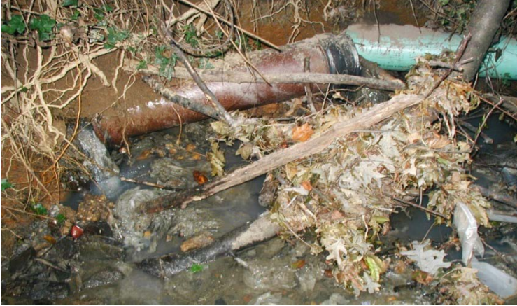
Streambank erosion can cause infrastructure damage to sewer pipes, leading to untreated sewage leaking into local streams.
