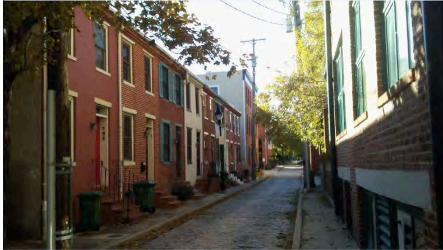
Figure 3: Two-and-a-half story houses with high basements (Photo courtesy Holly Simmons)
