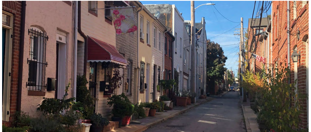
South Chapel Street, Fells Point (photograph courtesy Meagan Pickens)
