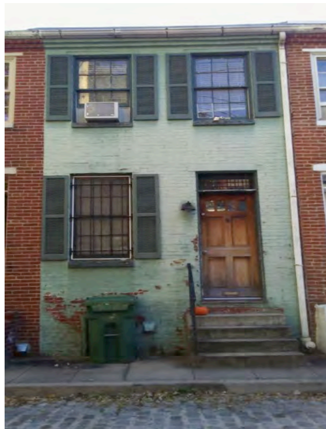
Figure 4: Brick cornices, 6 over 6 sash windows with a larger first floor window, painted brick facade with a transom over the door (Photo courtesy Holly Simmons)
