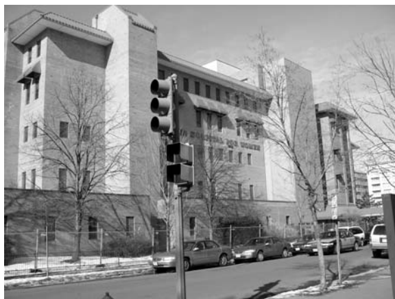
Figure 66: Current condition of west side of 24 th street
