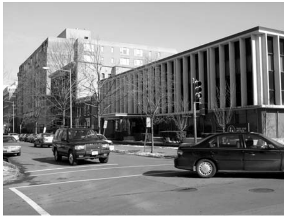
Figure 65: Current Condition of east side of 24 th street.
