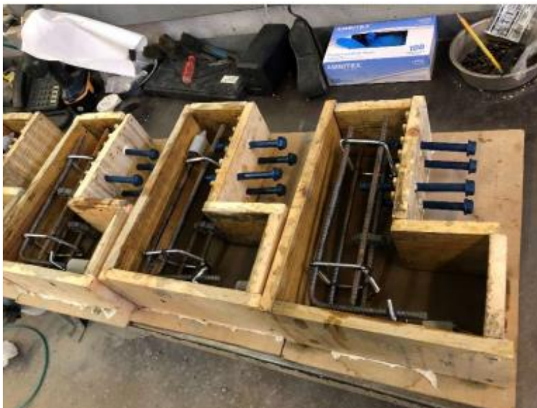
Figure 21: L-shaped underlay half formwork with anchors in place prior to concrete pouring
