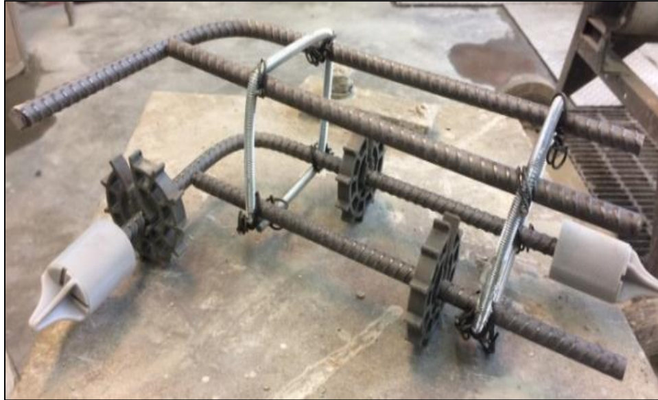
Figure 18: Reinforcement cage for the L-shaped halves
