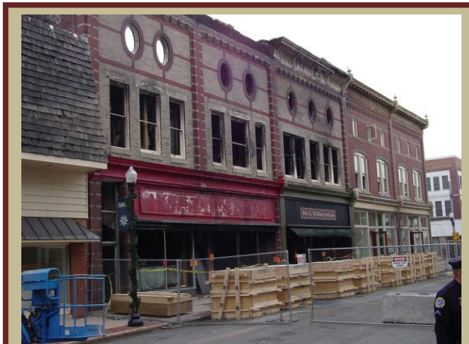
In January 2008, these two historic buildings in downtown Cambridge were gutted by a fire. Renovation of the buildings is subject to pending Community Legacy requests.
