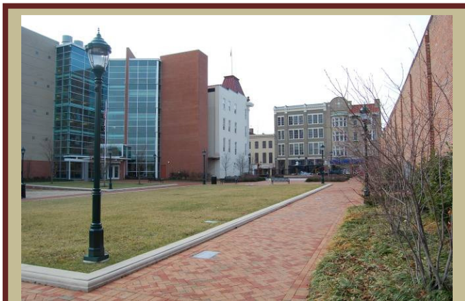
In Hagerstown, Community Legacy funding supported the demolition of the McCrory's building and creation of a community park. The project was conducted at the same time adjacent renovations brought the University System of Maryland to downtown Hagerstown.
