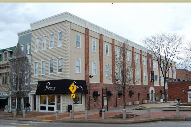
The Locust Lane pocket park in Westminster was initially funded through the Community Legacy program. Additional funding from the Neighborhood BusinessWorks program and private investments helped revitalize the surrounding community.
