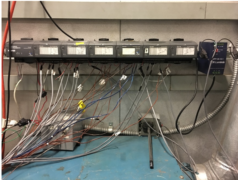
Figure 18: NI Data Acquisition Modules of the Outdoor Unit
