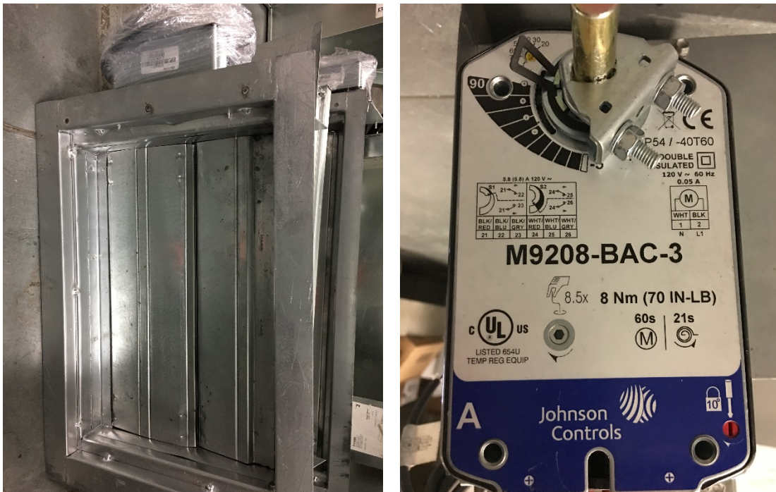
Figure 14: Air Damper with Electrical Actuator
