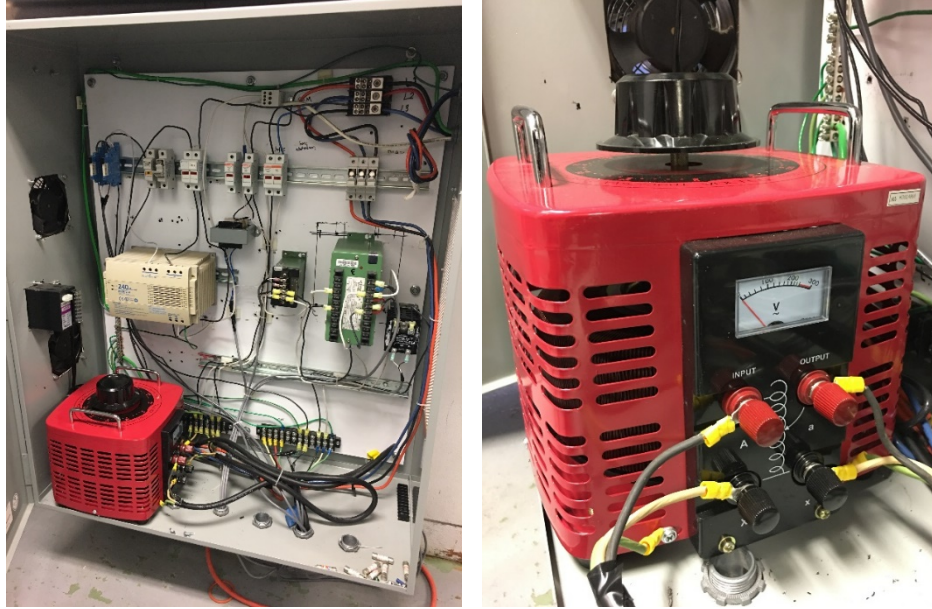
Figure 12: Overview of the Electric Box and the Variac for Outdoor Unit Power Supply
