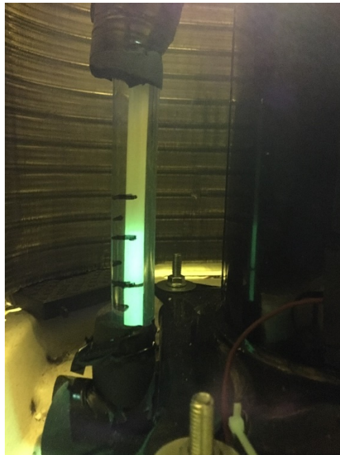
Figure 32: Compressor Oil Level under UV Light
