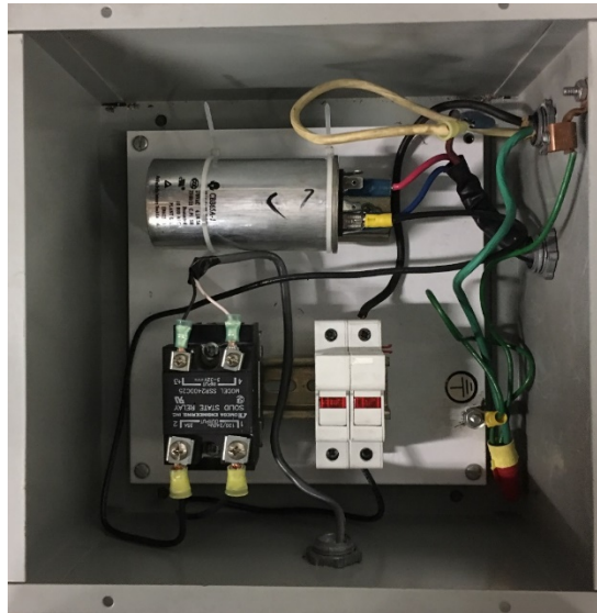
Figure 16: Electrical Box to Control the Recovery Compressor
