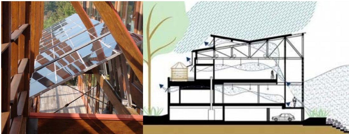
Figure 64: Philip Merrill Environmental Center- South Wall PV Panels for onsite energy production, Source theregeneration https://www.flickr.com/photos/theregeneration/2917294886 (accessed November 25, 2017).
