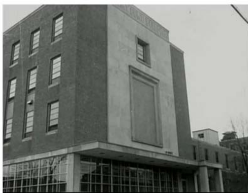
EXTERIOR OF JIMMY FUND BUILDING
