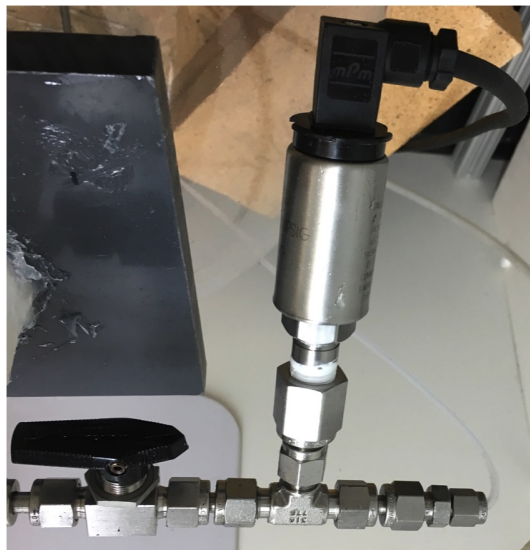
Figure 2.7: Valve installed to protect the pressure transducer
