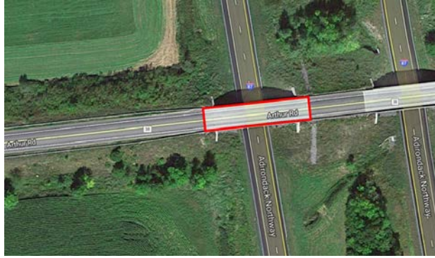
(a) Aerial view of the bridge site
