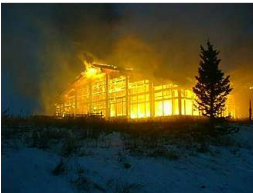
Figure 1: Two Elk Lodge in flames. Used with permission of the Vail Fire Department.
