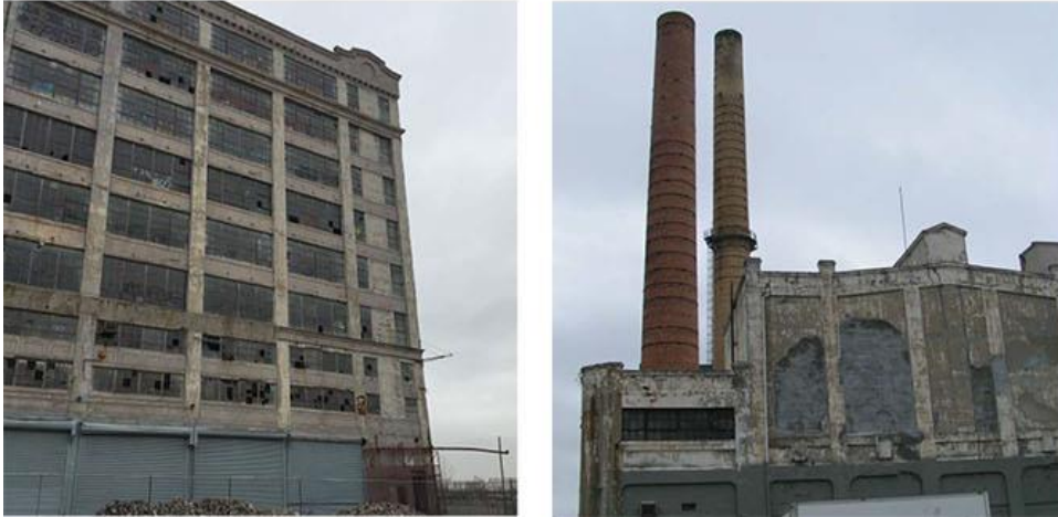
Figure 44: Abandoned Industrial Buildings Near Site Image by Author
