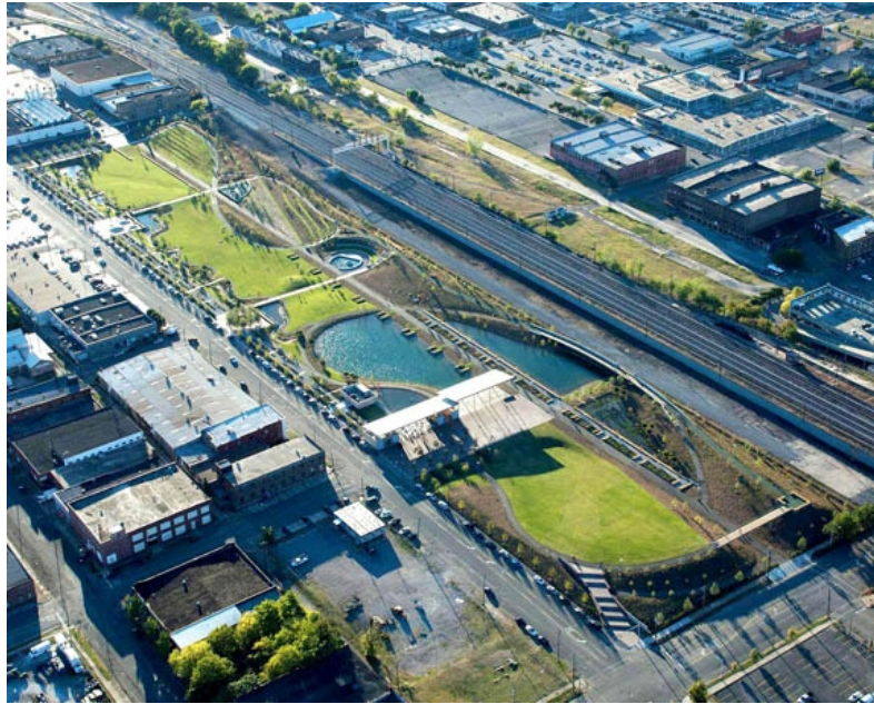
Figure 36 - Railroad Park, Birmingham, AL, aerial view. Source: t Islandarch.com
