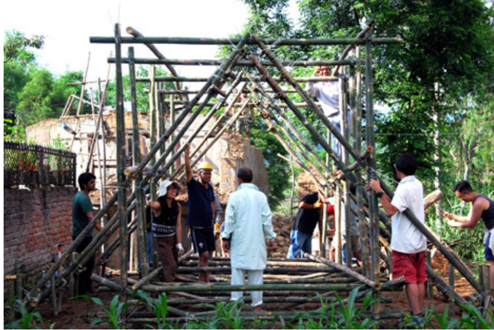
Figure 37 Volunteers working on the Shelter 114
