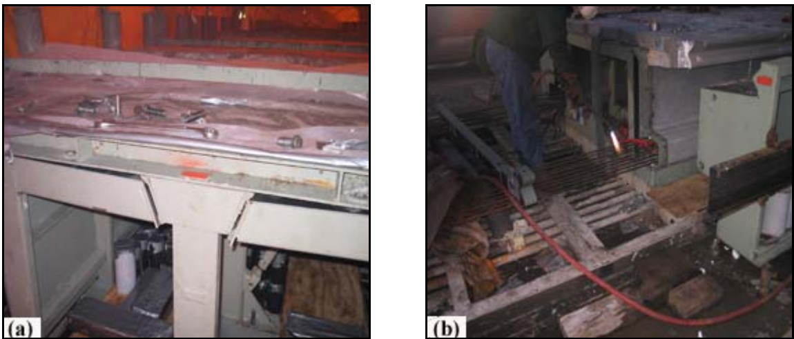
Figure 4.4 (a) Inner Forms Released and (b) Prestressing Strands being Cut.
