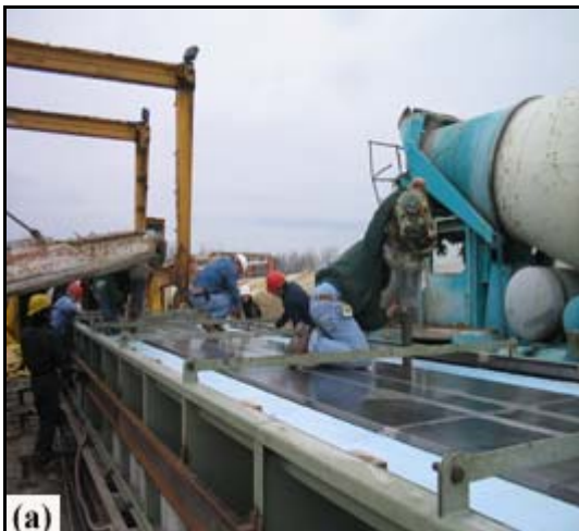
Figure 4.3 Placing UHPC
