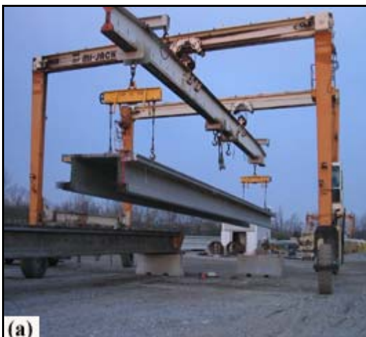
Figure 4.5 (a) Girder being Lifted and (b) Girder after it was Blocked.
