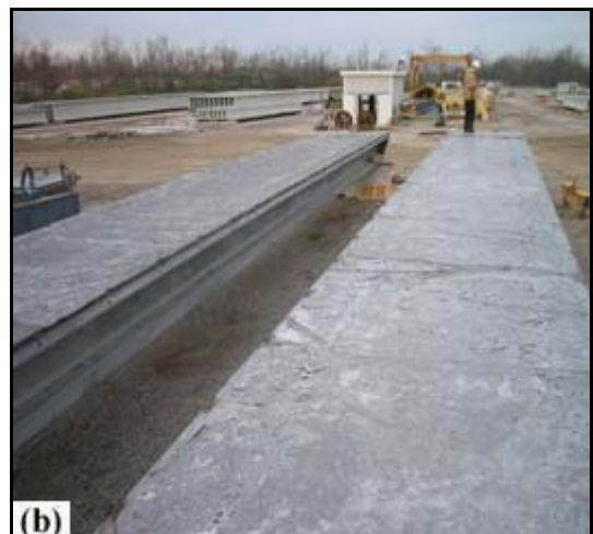
Figure 4.5 (a) Girder being Lifted and (b) Girder after it was Blocked.
