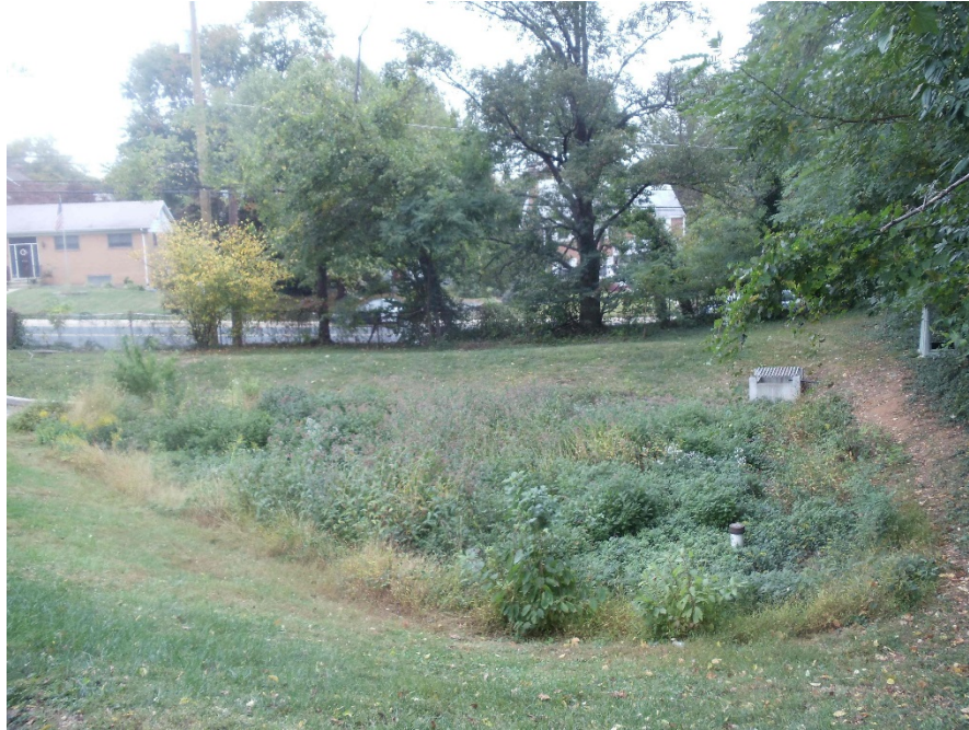
Figure 3.1 The study bioretention cell located in Silver Spring, Montgomery County, Maryland; (a) August 2006, five months after installation; (b) June 2009, with prominent species delineated; (c) October 2013, at the time of this study.
