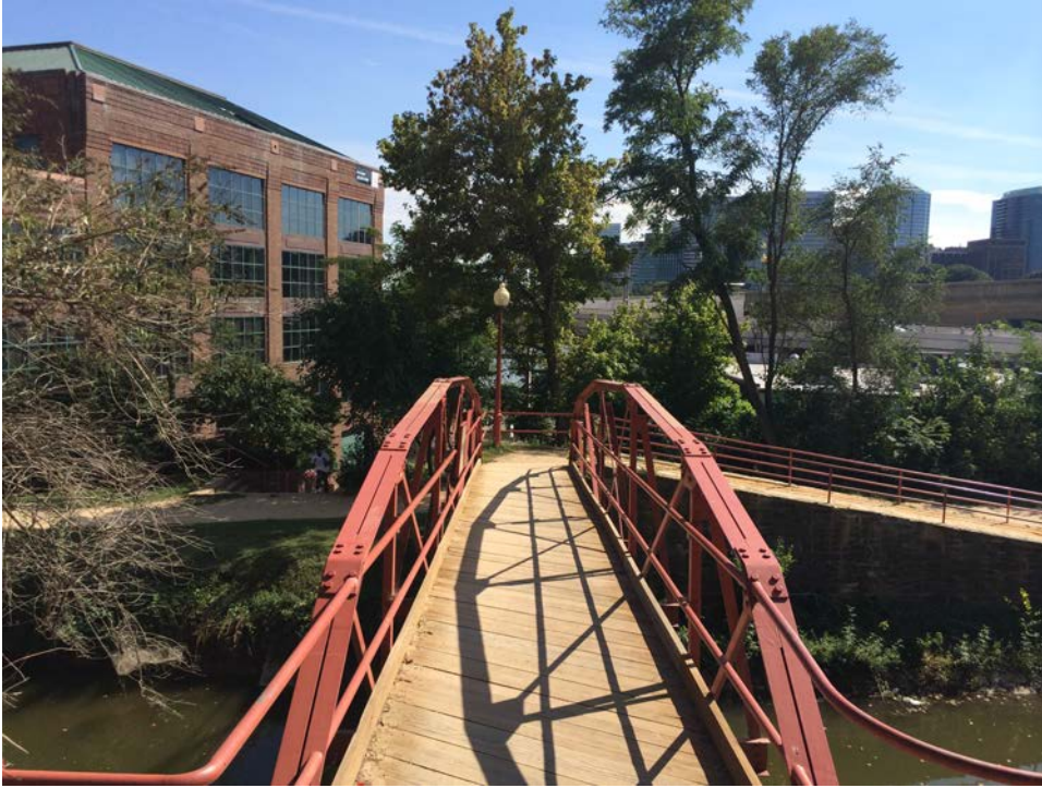
Figure 19: Transition 2 - 34 th Street bridge crossing
