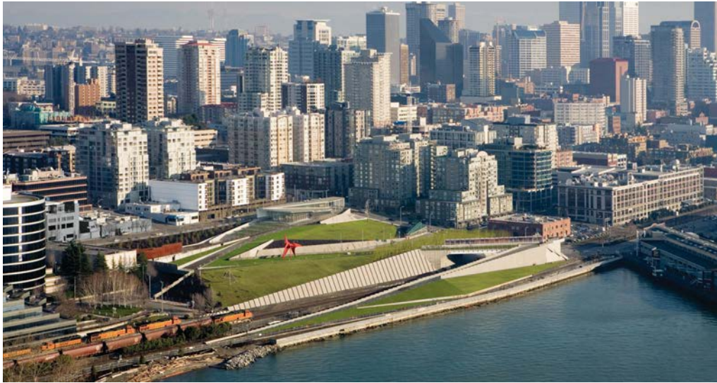
Figure 32: Aerial view of Olympic Sculpture Park
