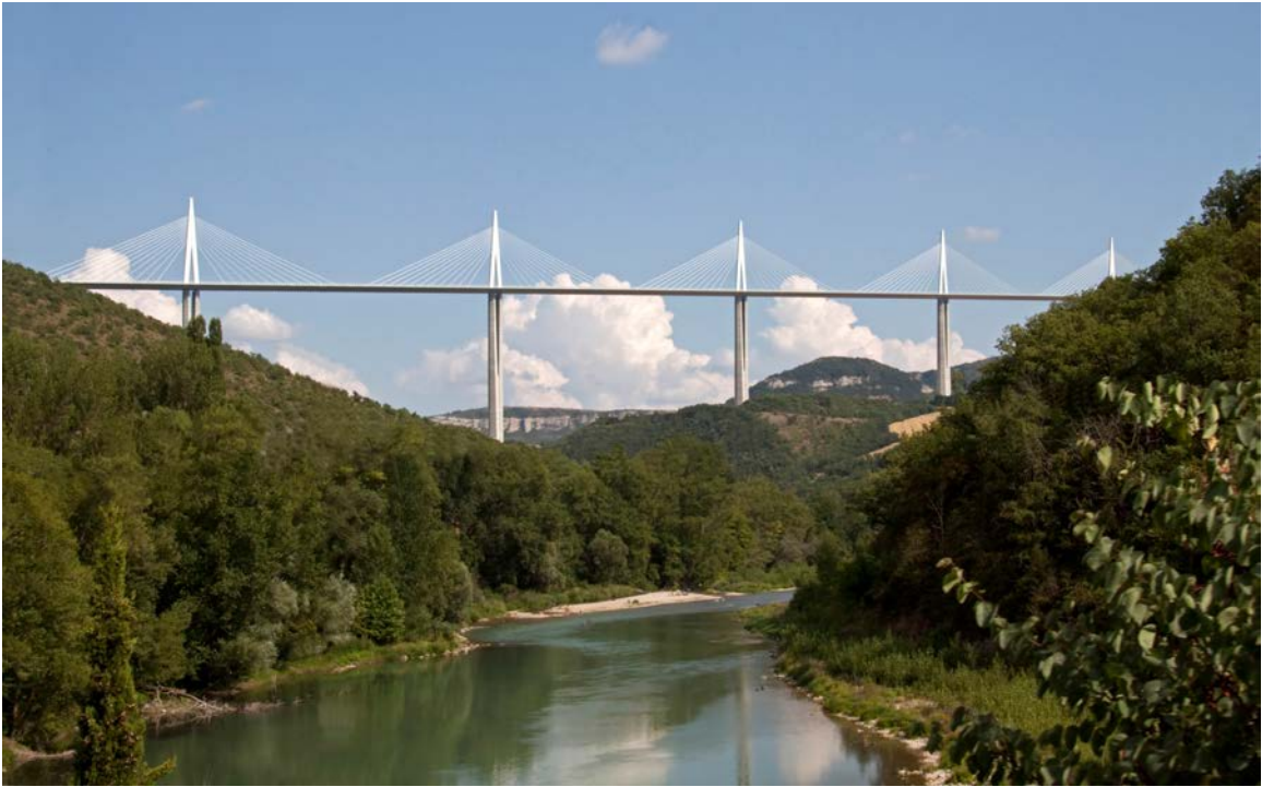
Figure 26: Millau Viaduct over the River Tarn
