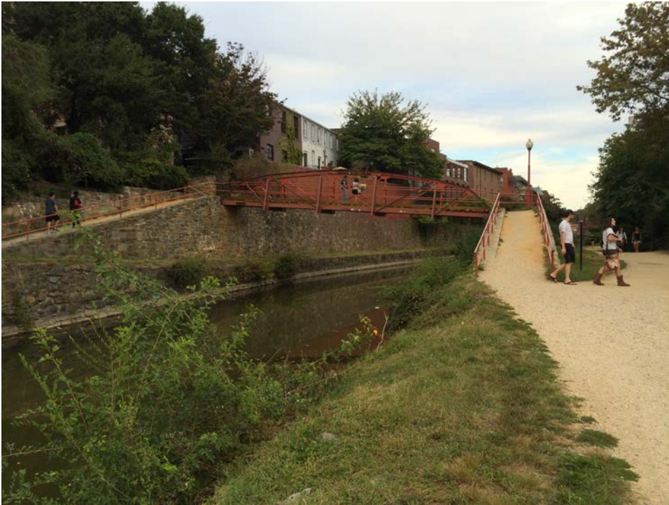
Figure 20: Transition 3 - Facing east along canal towards bridge
