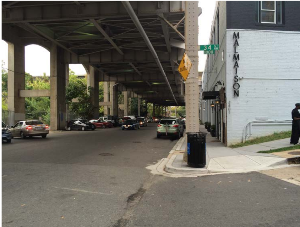
Figure 22: Transition 5 - Underneath Whitehurst facing west
