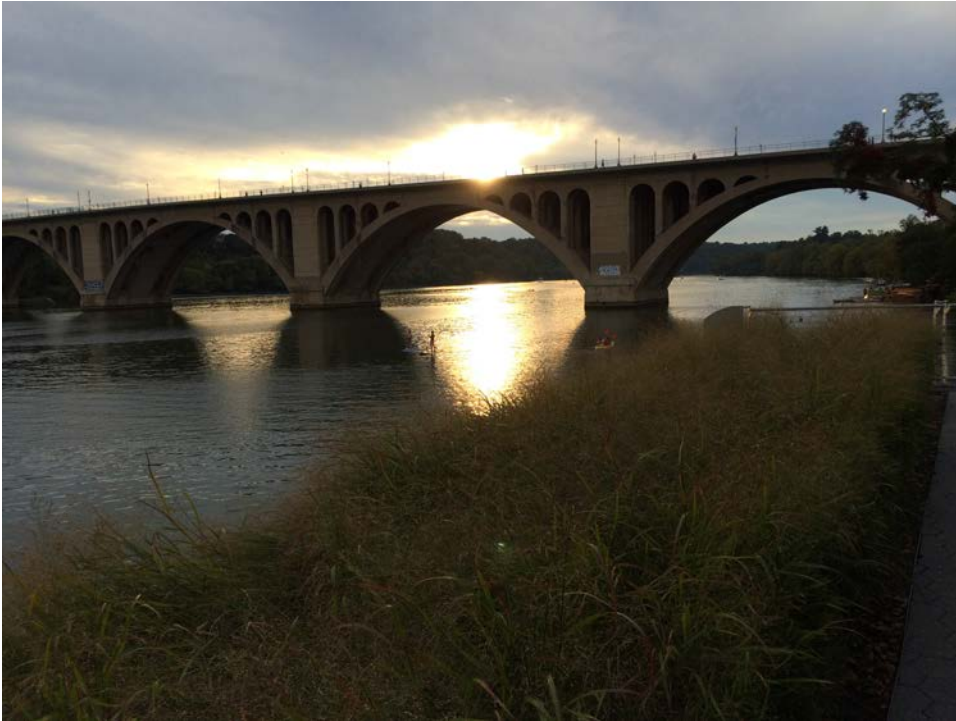
Figure 24: End - View of Key Bridge
