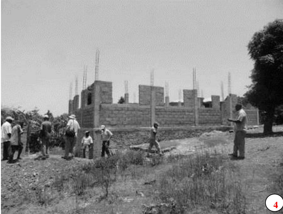
Figure 33: Facing towards front of building (Author)
