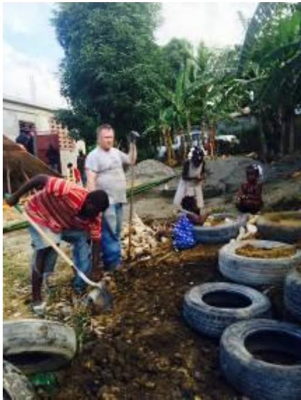
Figure 71: Soil Transferred from Ground to the Tires (Author)
