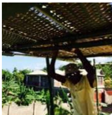
Figure 135: Attaching supports and coconut mat (Author)
