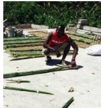
Figure 134: Assembling cross support (Author)
