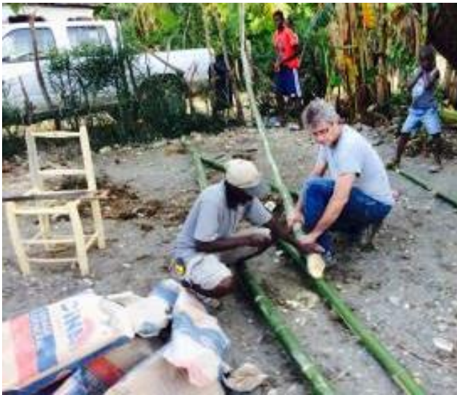
Figure 87: Carpenter Cuts Bamboo Lengths (Author)
