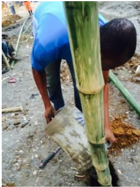
Figure 89: Volunteer pours concrete base (Author)
