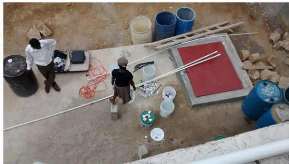
Figure 158: Cistern concrete top (Author)
