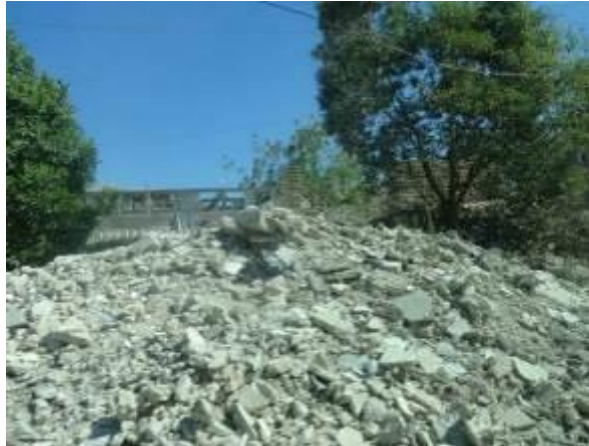
Figure 17: Concrete rubble (Author)
