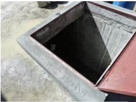
Figure 157: Cistern maintenance access (Author)
