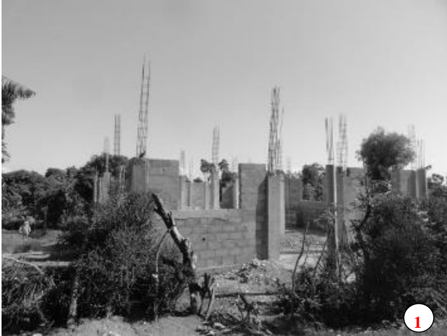
Figure 29: Front School Building from road (Author)
