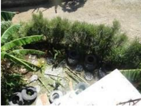
Figure 185: Prayer Garden During Construction (Author)
