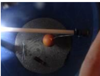
Figure 163: Float Valve Assembly (Author)
