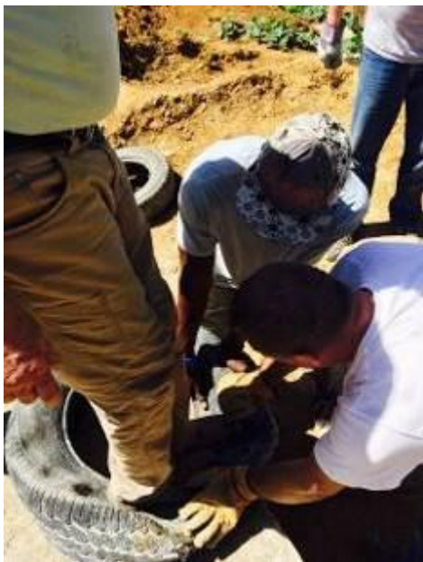
Figure 106: Volunteers work to invert tire (Author)
