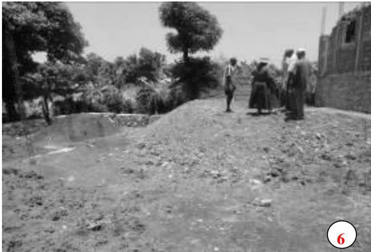
Figure 35: Soil Piles from Cistern Construction (Author)
