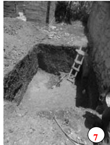
Figure 36: Cistern Under Construction (Author)
