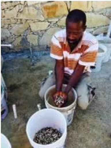
Figure 168: Washing Gravel (Author)
