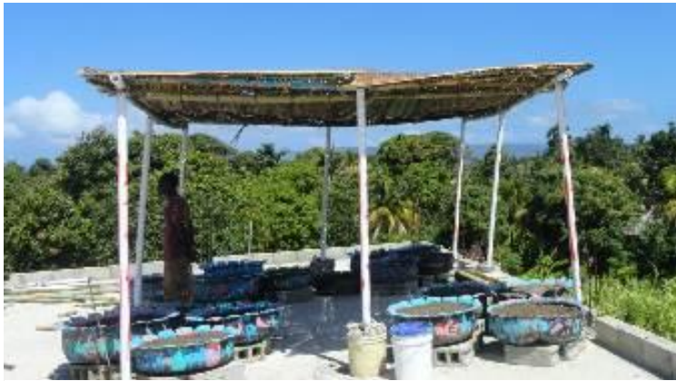
Figure 139: Finished shade structure (Author)
