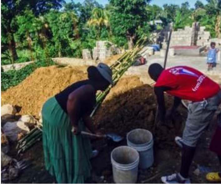
Figure 85: Volunteers Moving Soil in 5 gallon buckets (Author)
