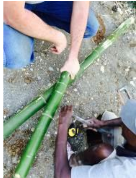
Figure 88: Haitian Carpenter Latches the Bamboo
