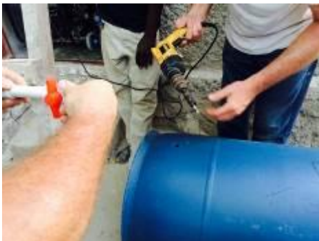
Figure 170: Volunteers Install Flow Valve (Author)
