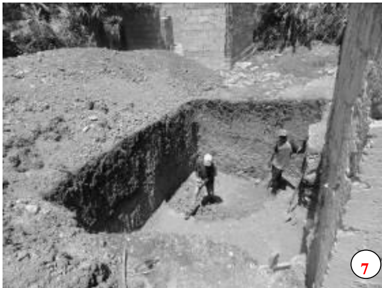
Figure 37: Workers Dig Cistern (Author)
