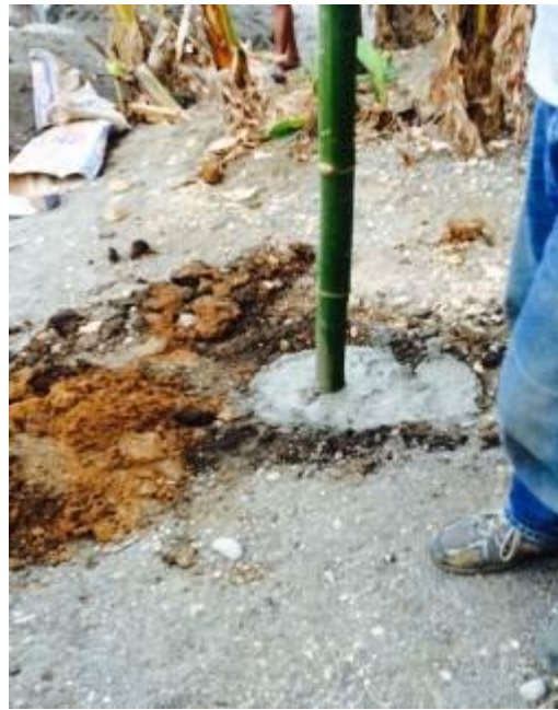
Figure 90: Concrete base of goal post
