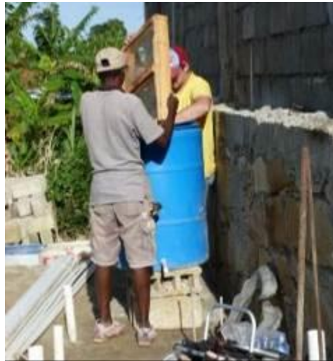
Figure 169: Adding Gravel to Filter (Author)
