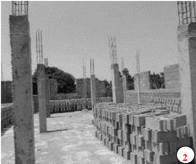
Figure 31: Support Columns (Author)
