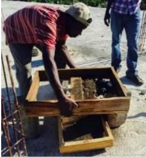
Figure 165: Sifting of Sand and Gravel (Author)
