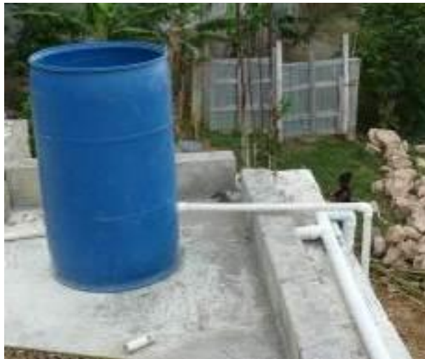
Figure 160: Pressure Barrel and Drain Pipes (Author)
