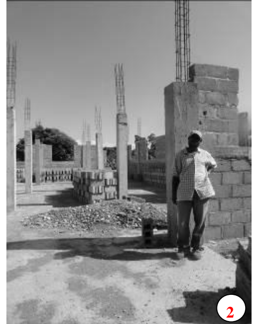
Figure 30: Entrance to front building (Author)
