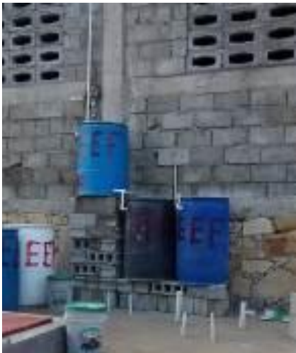
Figure 159: Slow sand filter system (Author)
