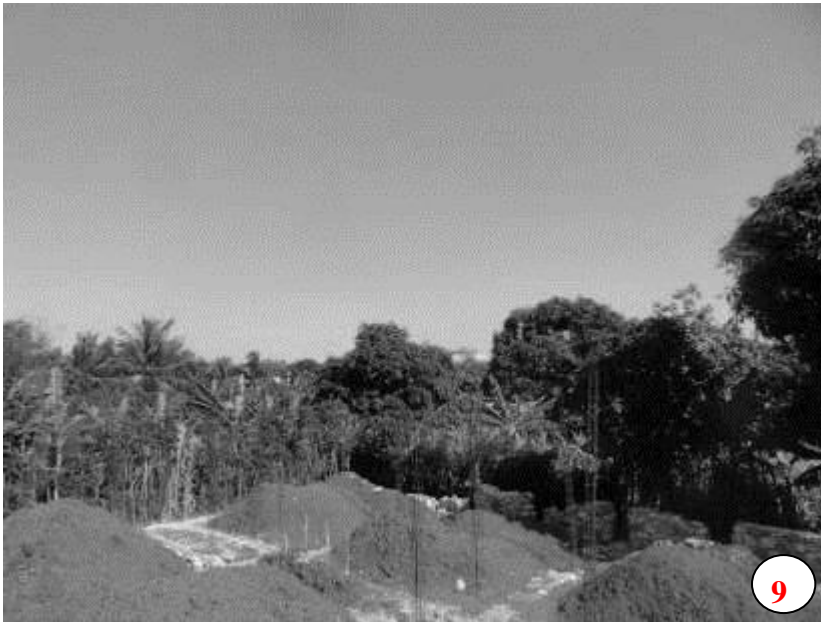
Figure 40: Rear School/Church Building Foundation
