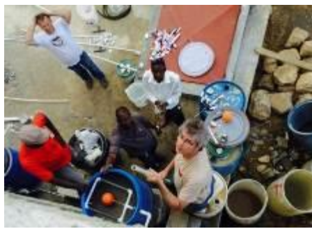
Figure 162: Above View of Float Valve and top diffuser (Author)
