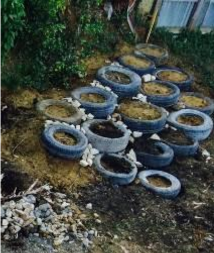
Figure 76: Layout of amphitheater during construction (Author)
