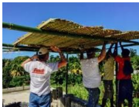
Figure 136: Attaching coconut mat (Author)
