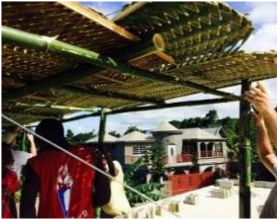
Figure 137: Structure supports (Author)
