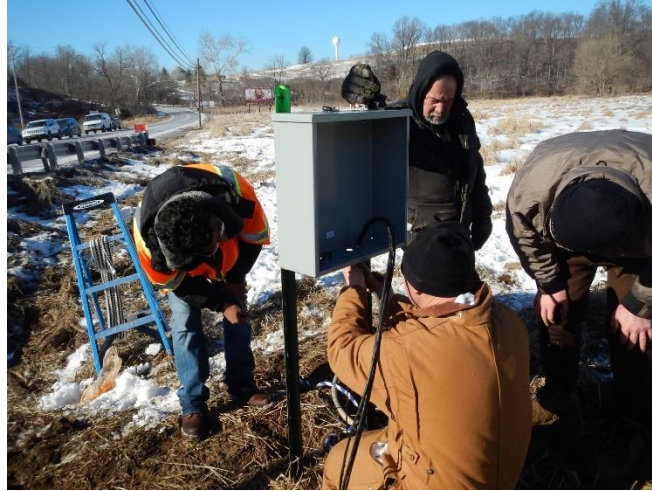
Figure 47. Electrical box for storing DAQ and electrical components for the second installation
