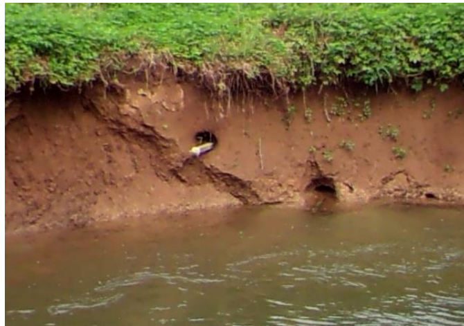
Figure 48. Residual cove formed from drilling
