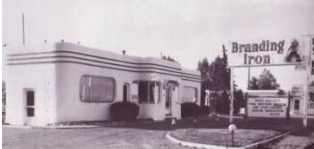
Figure 11: The Streamline Moderne Branding Iron Motel (From “Motels,” University of Vermont , accessed March 26, 2014, http://www.uvm.edu/landscape/dating/roadside_architecture/motels.php ).
