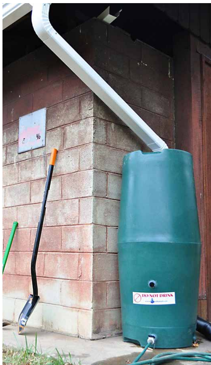
Rain barrels conserve water by collecting rain water from roofs. Rain barrels can then be used for watering gardens and washing cars.
