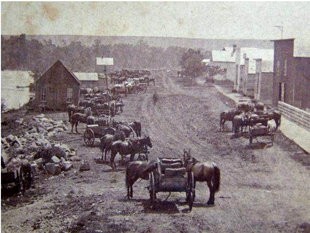
Figure 4. Downtown Granite Falls, late 19th century ( Source: Granite Falls Historical Society, used with permission ).
