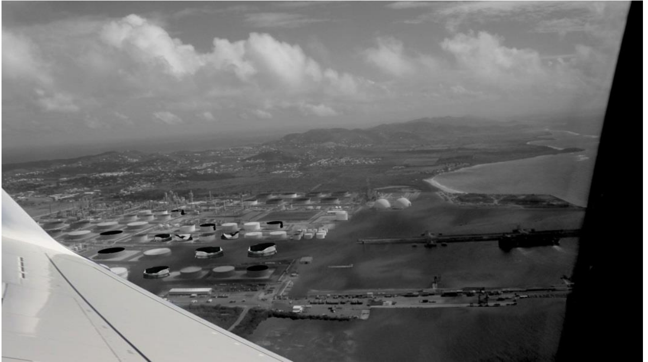
Figure 11: View of Hess Oil Refinery current conditions after a hurricane [Abraham]
