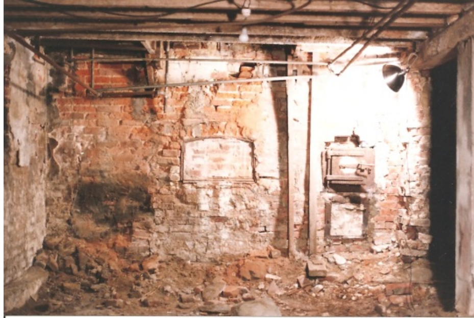
Figure 6.3. Photo showing the end wall of the basement at 30 Cornhill Street with ovens, following the plaster removal during construction in 1978 (Photo courtesy of the Davisson family).
