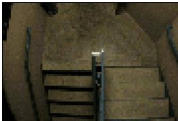
Figure 3-1: Typical Camera View in Building 4 [32]
